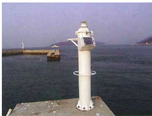
Figure 6.5.3 Example of Light Beacon (Straight Light Beacon 5m Type)
