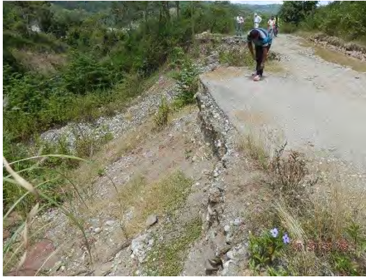
Photo 2.21 Condition at 125.4 km point
