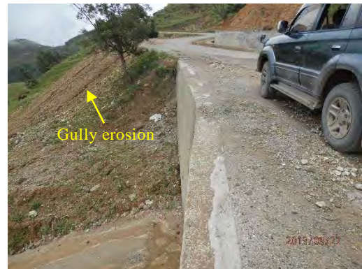
Photo 2.12 Condition at 81.4 km point
