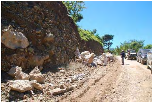
Photo 2.17 Condition at 103.6 km point
