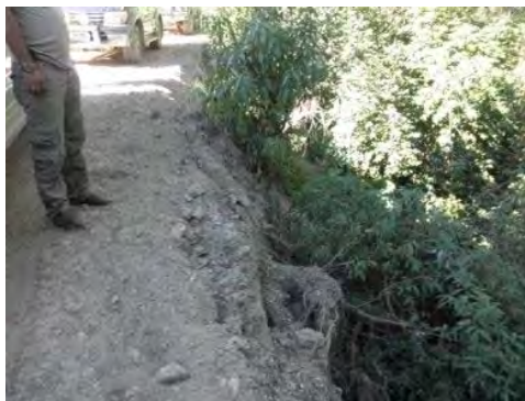
Photo 2.13 Condition at 83.1 km point
