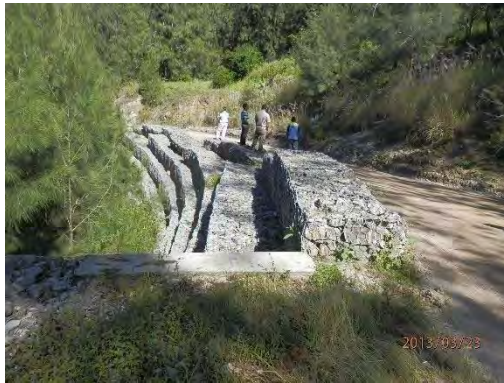
Photo 2.15 Condition at 91.2 km point
