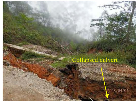
Photo 2.9 Condition at 27.8 km
