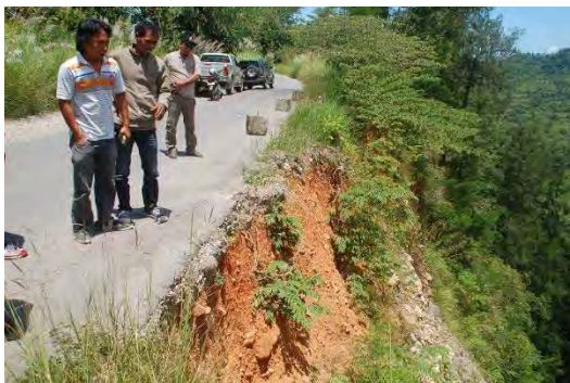
Photo 2.19 Condition at 114.5 km point
