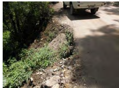
Photo 2.14 Condition at 85.8 km point
