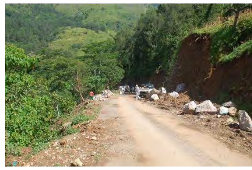
Photo 2.18 Condition at 103.6 km point
