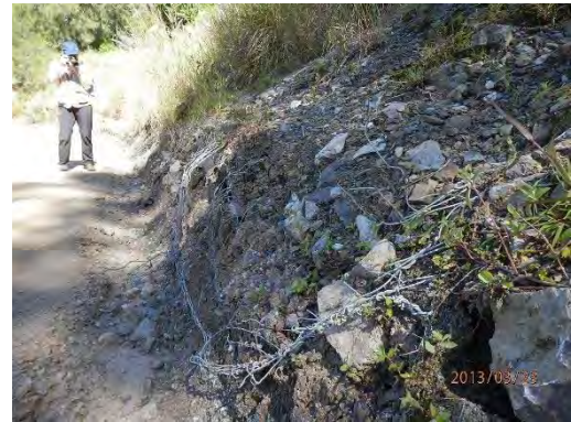
Photo 2.16 Condition at 91.2 km point
