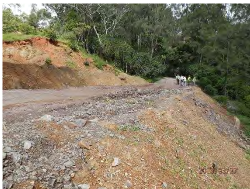
Photo 2.10 Condition at 68.3 km
