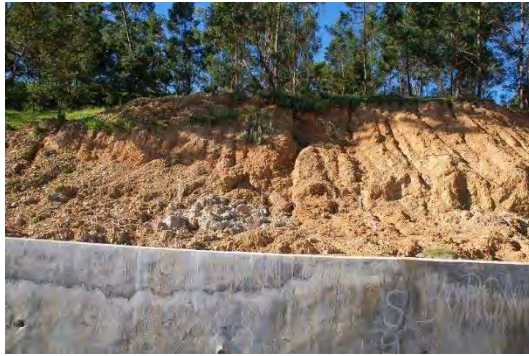
Photo 2.11 Condition at 81.4 km point
