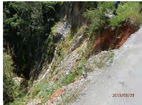
Photo 2.20 Condition at 114.5 km point
