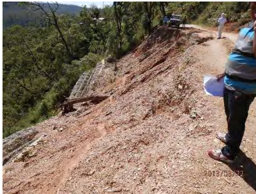
Photo 2.8 Condition at 27.7 km
