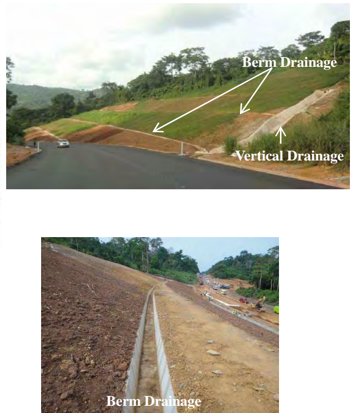
写真4 Vertical Drainage /Berm Drainage
