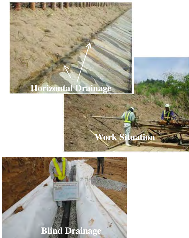
写真3 Horizontal Drainage /Blind Drainage
