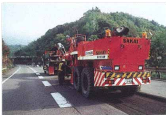
Cutting and loading of the pavement waste
