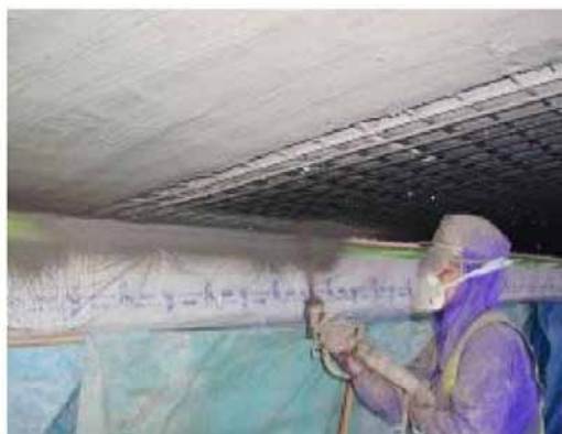
Figure 2.4-12 Pneumatically Applied Polymer Cement Mortar
