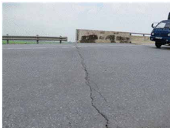
Planar cracking Reflective cracking (develops into a structural failure) (at the end of an approach slab)
