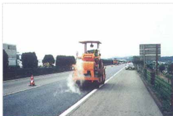
Primary compaction by a road roller
