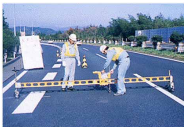
Measuring rutting using a transverse profile meter
