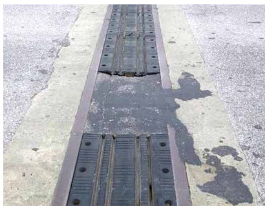
Figure 2.4-1 Temporary Filling with Bituminous Mixtures
