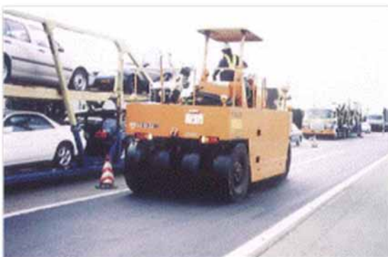
Secondary compaction by a tire roller
