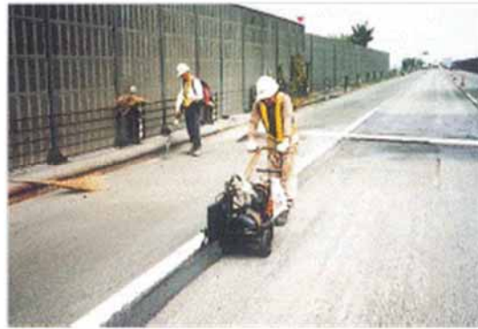
Tack coat (treatment at the edge)
