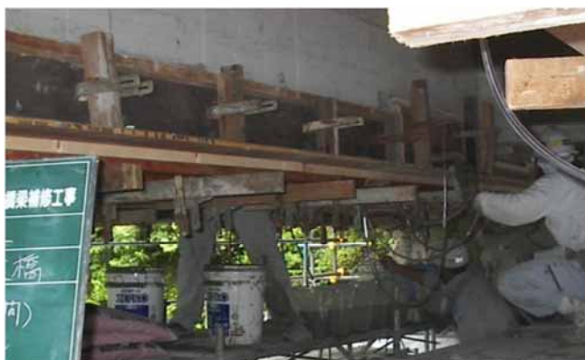
Figure 2.4-11 Filling of Non-Shrinkage Mortar
