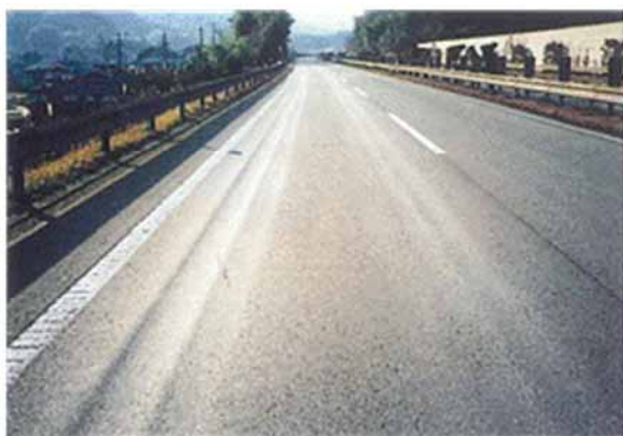
Rutting caused by the flow of asphalt mixture Rutting caused by friction
