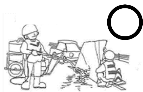
The spreading of materials is prevented with concrete panels.
