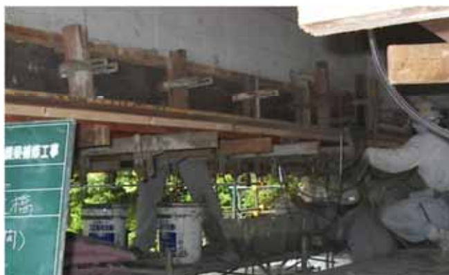
Figure 2.4-11 Filling of Non-Shrinkage Mortar
