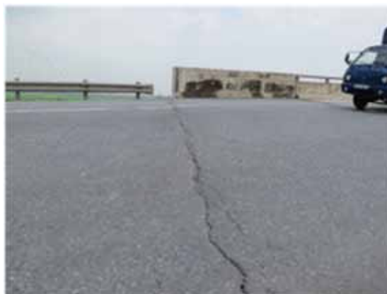
Planar cracking Reflective cracking (develops into a structural failure) (at the end of an approach slab)
