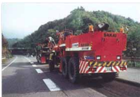
Cutting and loading of the pavement waste
