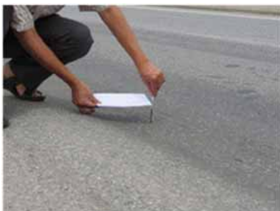
Rutting due to the flow of asphalt mixture cracking
