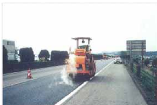
Primary compaction by a road roller
