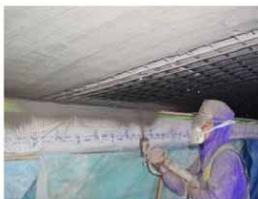
Figure 2.4-12 Pneumatically Applied Polymer Cement Mortar
