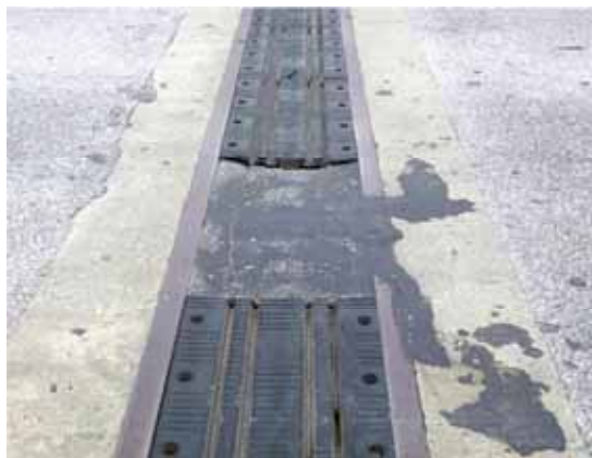
Figure 2.4-1 Temporary Filling with Bituminous Mixtures
