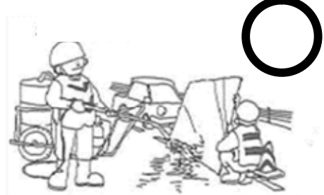
The spreading of materials is prevented with concrete panels.
