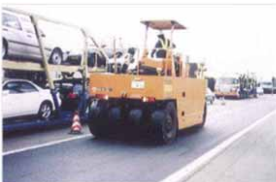
Secondary compaction by a tire roller
