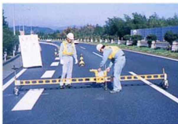
Measuring rutting using a transverse profile meter
