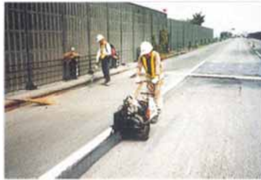
Tack coat (treatment at the edge)
