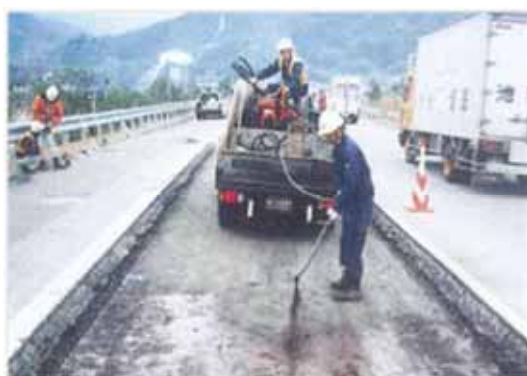
Laying a prime coat on a lower base course using an engine sprayer.
