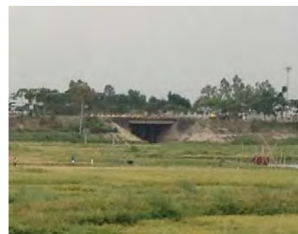
Photo: Difference in elevation between planned site and National Highway
