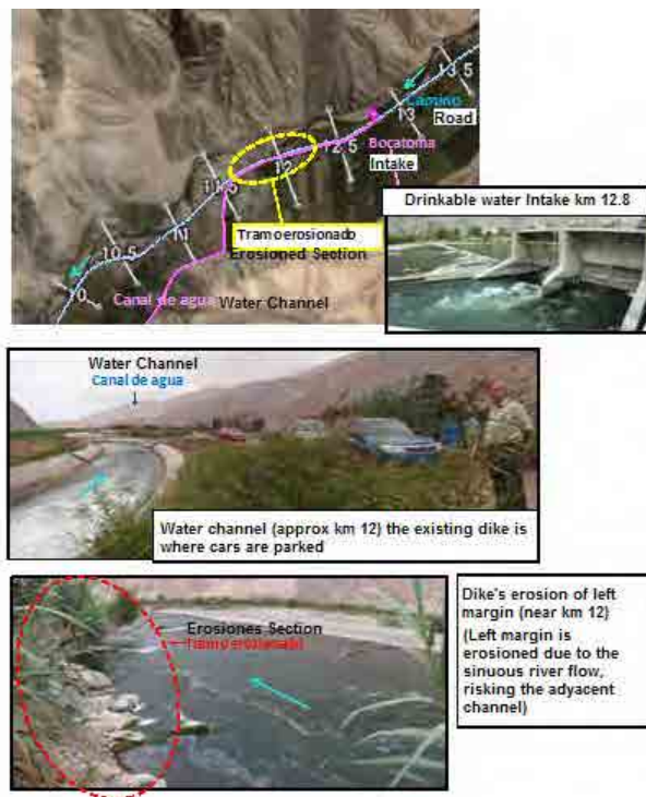
Figure 3.1.6-4 Local conditions related with Challenge 2 (Camana River)
