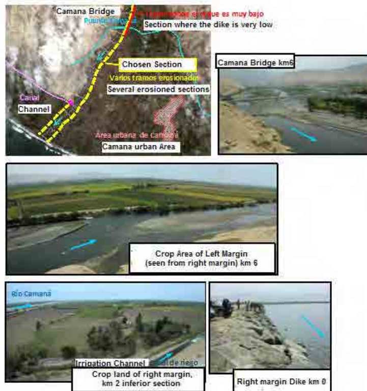
Figure 3.1.6-3 Local conditions related with Challenge 1 (Camana River)
