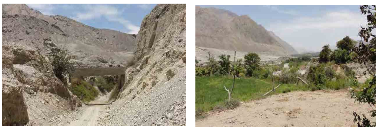
Figure 3.1.8-14 Situation of the sediment deposition in the San Francisco river (obstruction of irrigation channels due to the disaster. The walls of the highway are the soil and sand sediments at that time)
