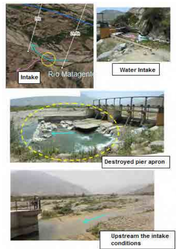
Figure 3.1.6-3 Local conditions related with Challenge 2 (Chíncha River)
