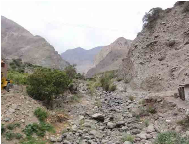
Figure 3.1.8-8 Andesitic and basaltic soil collapsed
