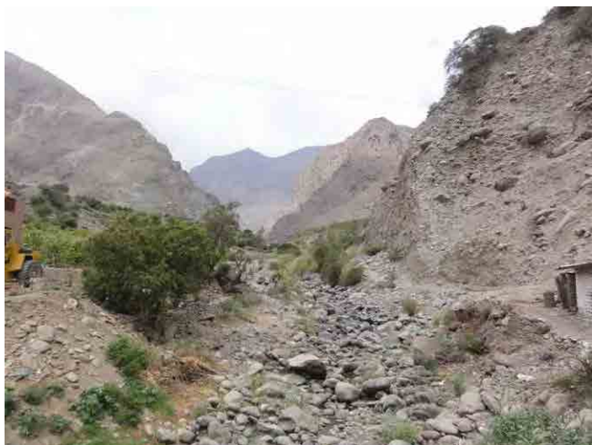
Figure 3.1.8-8 Andesitic and Basaltic lands collapse
