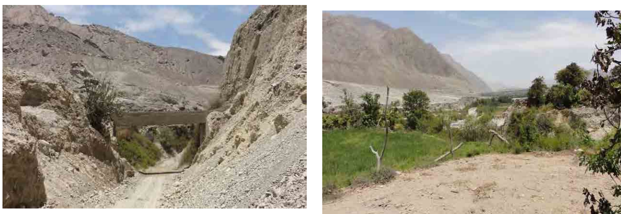
Figure 3.1.8-14 Situation of the sediment deposition in the San Francisco river (obstruction of irrigation channels due to the disaster. The walls of the highway are the soil and sand sediments at that time)
