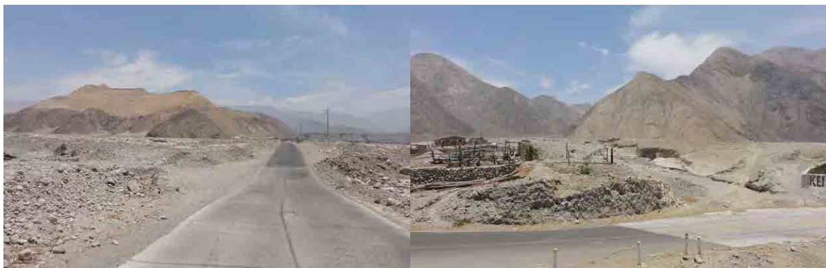
Figure 3.1.8-12 Rural (=local) highway crossing the Cosos river (in rainy season the sediments cover the rural highway, however, it is restored in a day)
