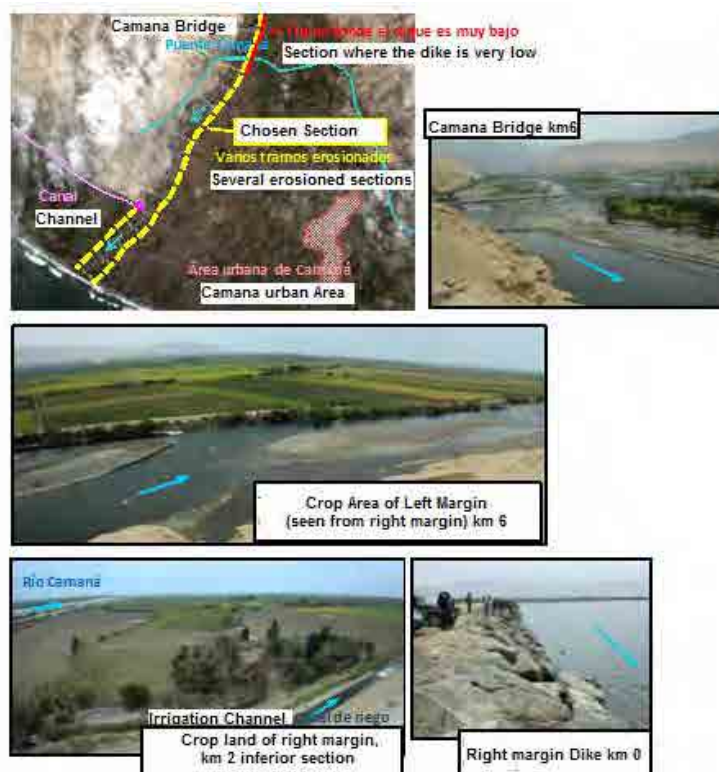
Figure 3.1.6-23 Local conditions related with Challenge 1 (Camana River)
