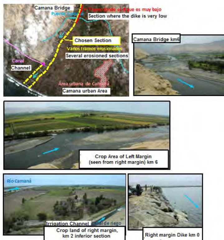
Figure 3.1.6-3 Local conditions related with Challenge 1 (Camana river)
