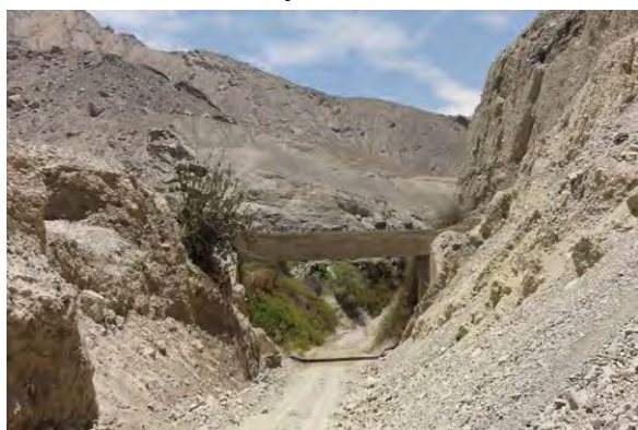
Figure 3.1.8-14 Situation of the sediment deposition in the San Francisco river (obstruction of irrigation channels due to the disaster. The walls of the highway are the soil and sand sediments at that time)
