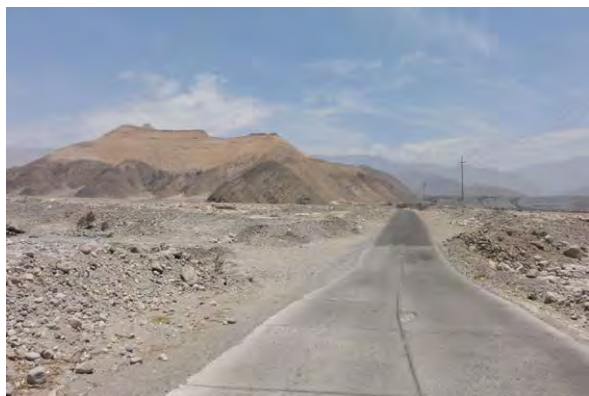
Figure 3.1.8-12 Rural (=local) highway crossing the Cosos river (in rainy season the sediments cover the rural highway, however, it is restored in a day)
