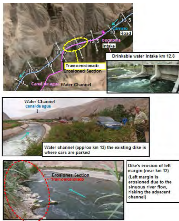
Figure 3.1.6-4 Local conditions related with Challenge 2 (Camana river)
