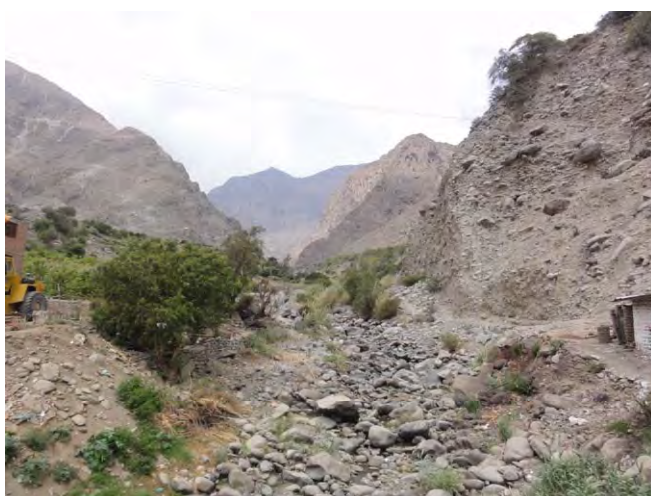
Figure 3.1.8-12 Andesitic and basaltic soil collapsed
