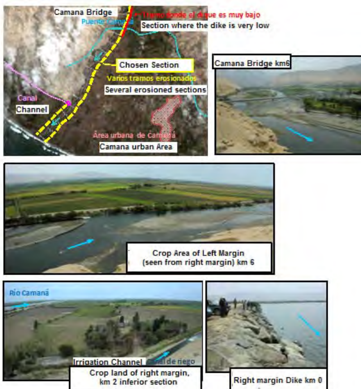
Figure 3.1.6-15 Local conditions related with Challenge 1 (Camana river)
