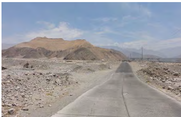
Figure 3.1.8-20 Rural (=local) highway crossing the Cosos river (in rainy season the sediments cover the rural highway, however, it is restored in a day)
