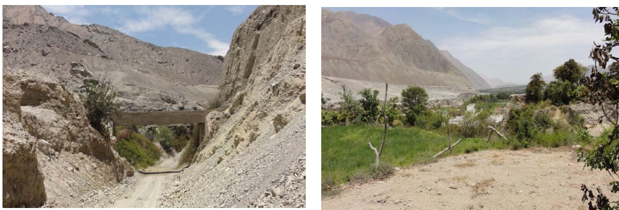
Figure 3.1.8-14 Situation of the sediment deposition in the San Francisco river (obstruction of irrigation channels due to the disaster. The walls of the highway are the soil and sand sediments at that time)
