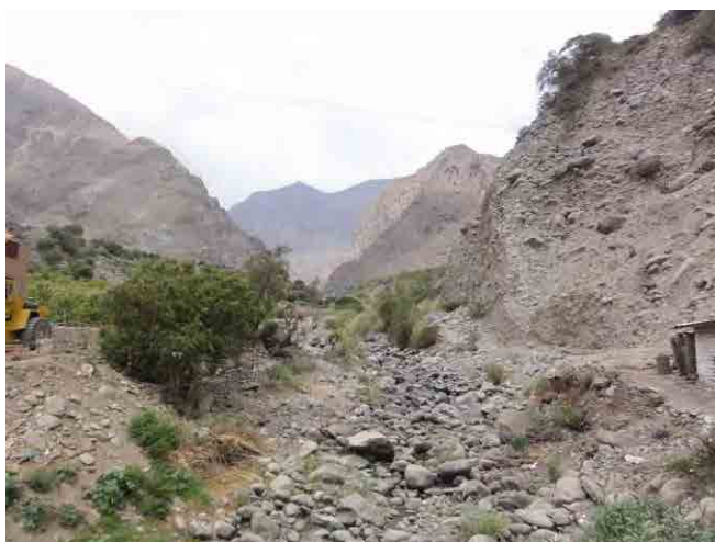
Figure 3.1.8-8 Andesitic and Basaltic lands collapse
