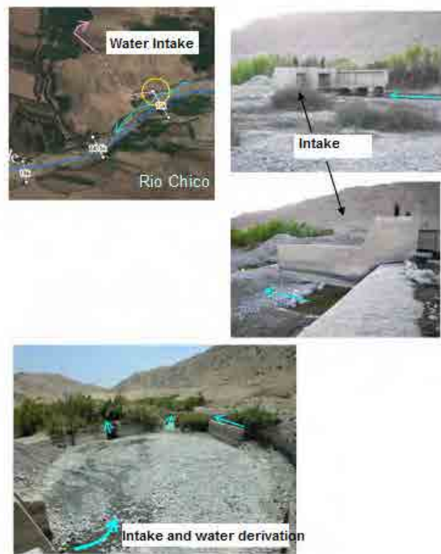
Figure 3.1.6-4 Local conditions related with Challenge 3 (Chíncha River)
