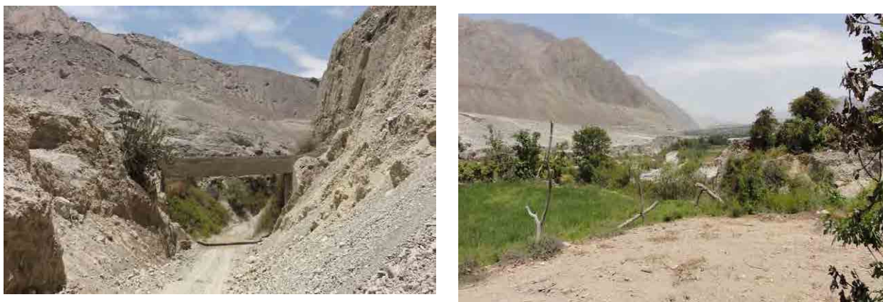
Figure 3.1.8-14 Situation of the sediment deposition in the San Francisco river (obstruction of irrigation channels due to the disaster. The walls of the highway are the soil and sand sediments at that time)
