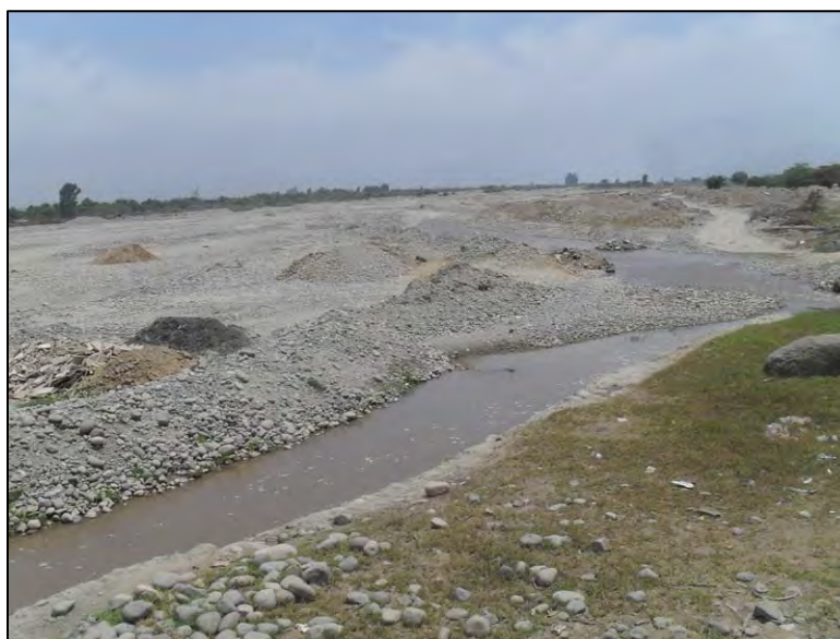
Figure 4.14 CAVERO Drainage Structure Constructed by the Area's Residents (Ma - 02)
