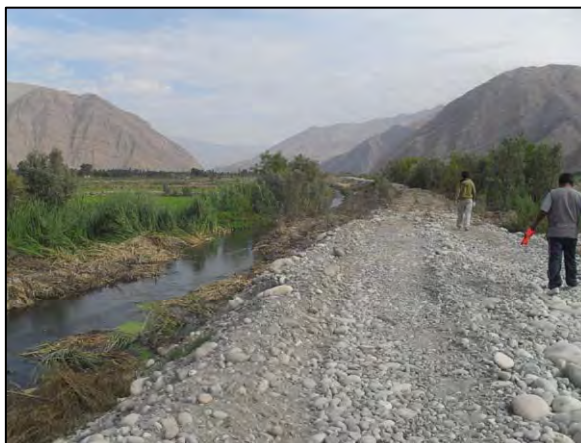
Figure 4.15 PAMPA BLANCA Drain Ditch (MC-05)
