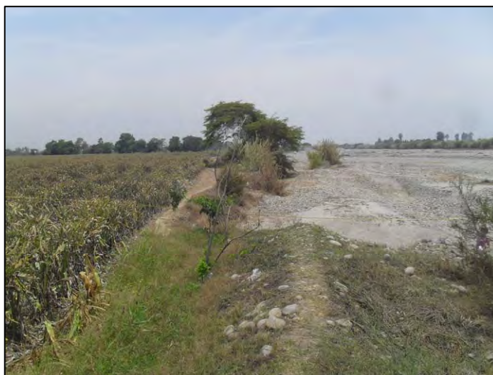
Figure 4.2 Dike without Revetment in Farmland/ Area along River/ Area under Production
