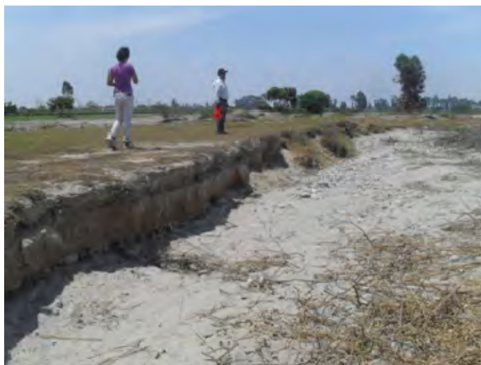
Figure 4.1 Dike without Revetment in Farmland/ Area along River/ Erosion Area
