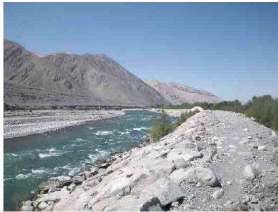
Figure 3.6 Dike in Majes-Camana River
