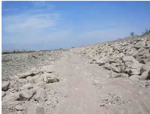
Figure 3.3 Revetment Works by Boulder near the River Mouth in Pisco River
