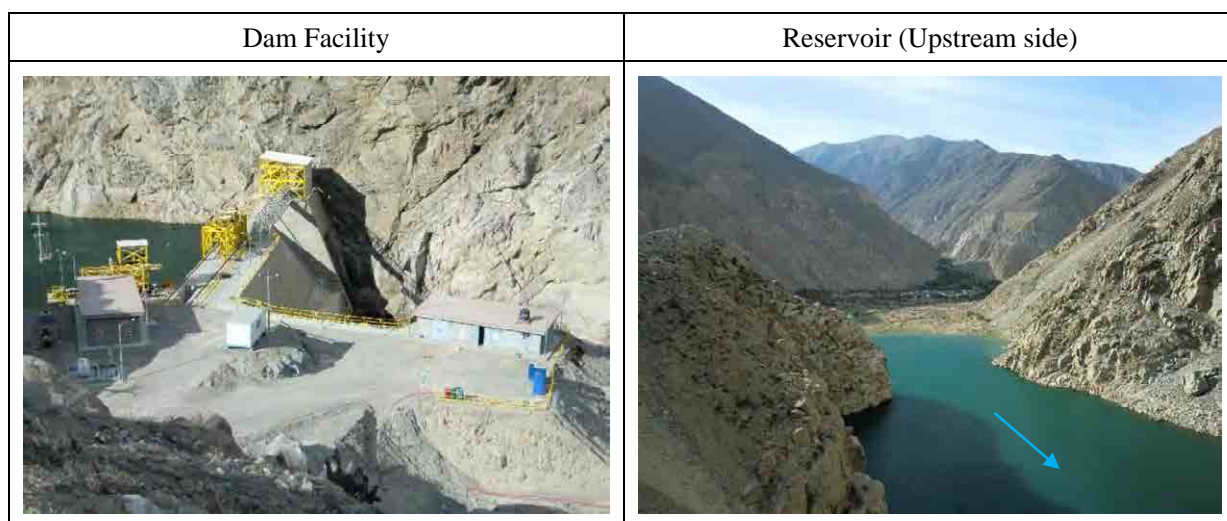
Figure 2.5 Overview of Plantanal Dam
