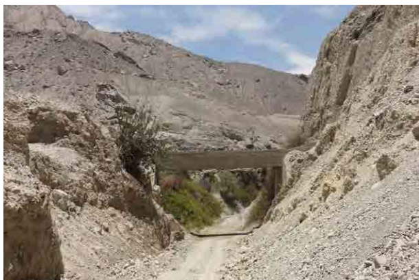
Figure 3.1.8-22 Situation of the sediment deposition in the San Francisco river (obstruction of irrigation channels due to the disaster. The walls of the highway are the soil and sand sediments at that time)
