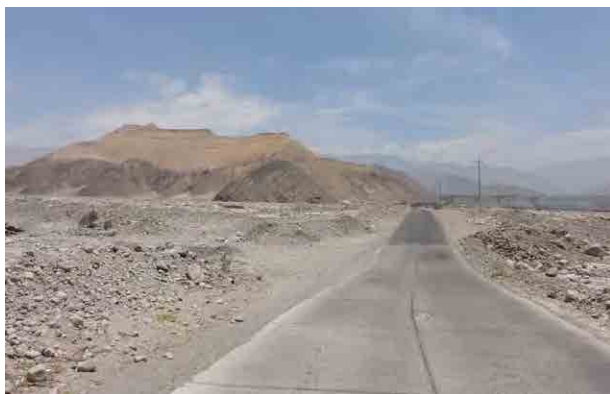
Figure 3.1.8-20 Rural (=local) highway crossing the Cosos river (in rainy season the sediments cover the rural highway, however, it is restored in a day)
