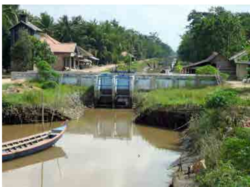
Secondary canal and gate
