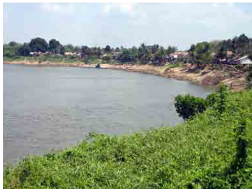
Musi mainstream river bank erosion (Kec. Lais)
