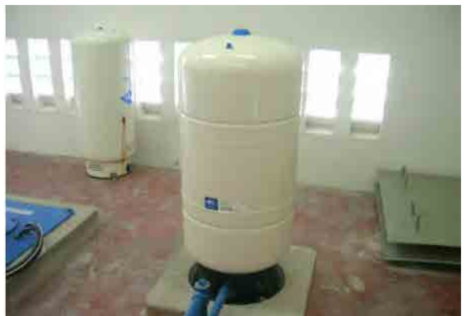
After rehabilitation Pressure tank: Pressure tank is replaced and used properly
