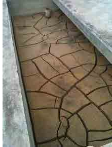
After rehabilitation Sludge Drying Bed Gravel and sand are filled, and sludge drying bed is functioning properly.
