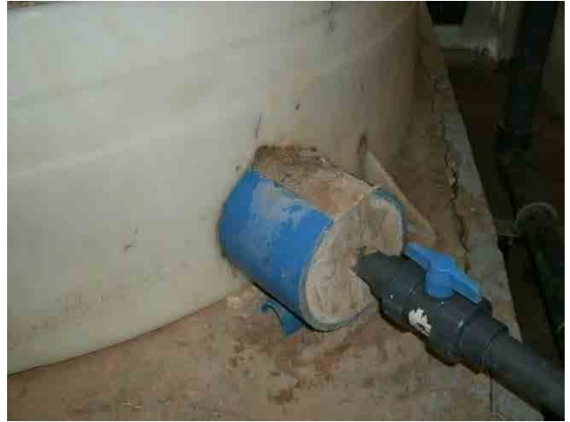
Chlorine tank: Leakage of chlorine solution has been repaired by WD.
