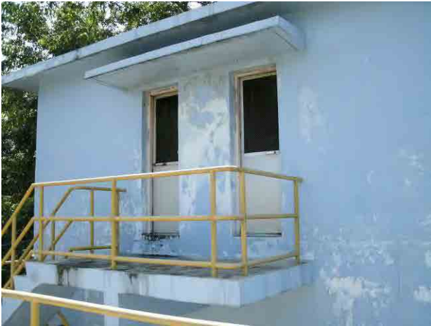
Aeration tower: Aluminum door installed by WD
