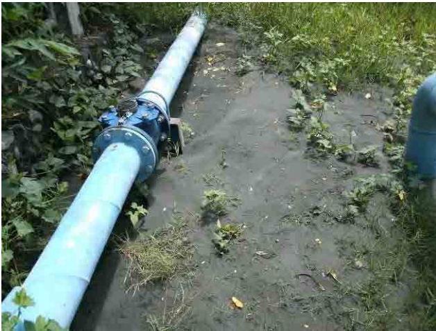
No.7 Well: Excess sand is pumped up.
