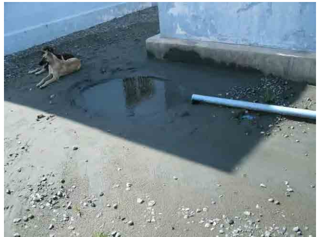
Sand separator: Sand is raised by pumping from the well.
