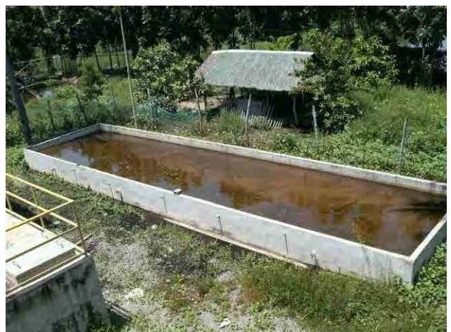
Sludge Storage basin: A sludge storage basin was constructed by WD for receiving the excess sludge.
