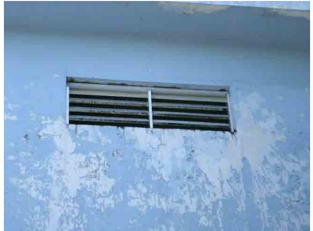
Aeration tower: Aluminum louver installed by WD
