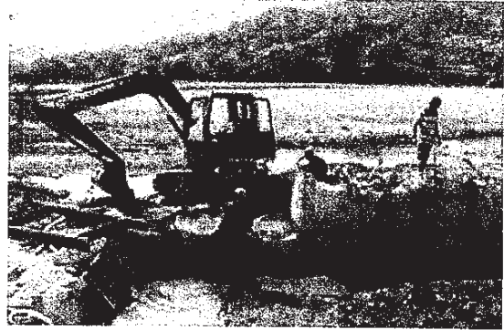
Gabion Installation at Intake for Dirimane
