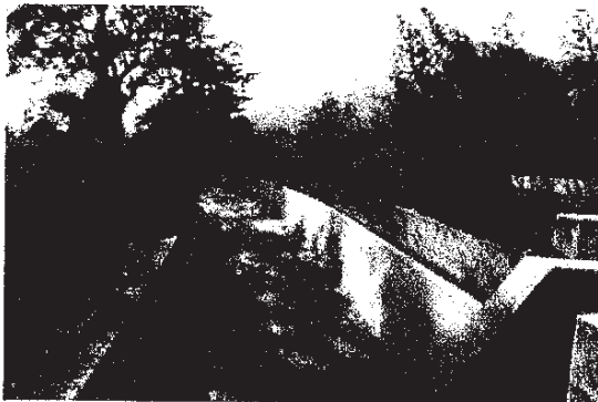
Spillway on the Main Canal/Laclo Irrigation Scheme
