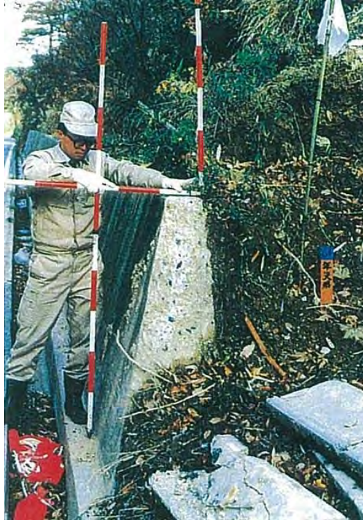
Photo2.2.15 Measuring cross-section of an existing structure
