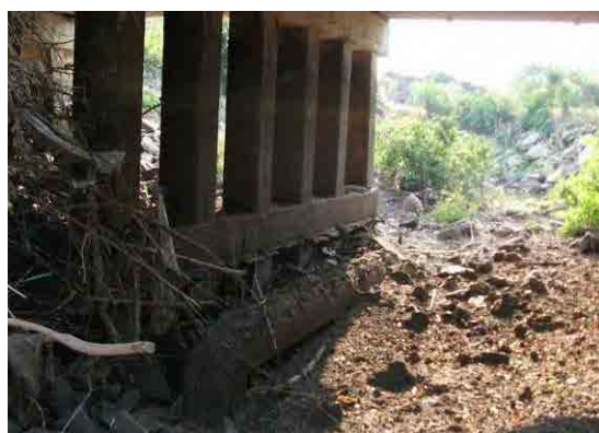
Lop Buri LB1030 - Br1. The riverbed around the pier was locally scoured and the pile heads have been exposed. Moreover, some floodwoods have still left on the pier upstream and disturbs the flow.
