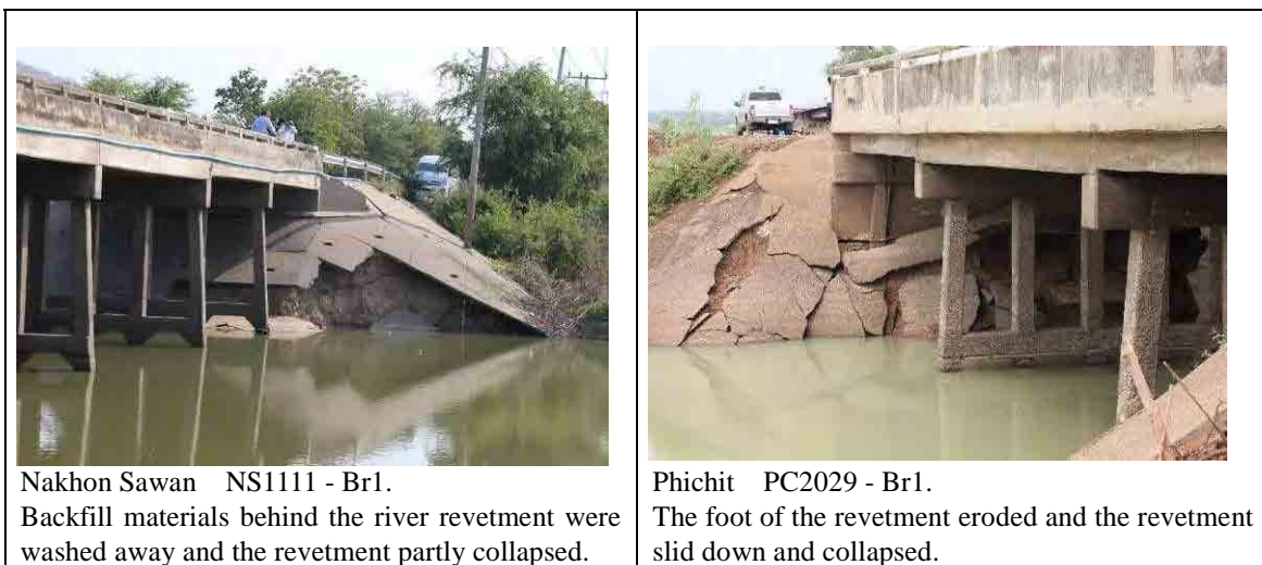
Photo 7.3.2 Damages / collapse of river revetments near abutments
