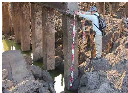
Lop Buri LB1030 - Br2. The pile heads are exposed. The scouring depth is about 2.5m.
