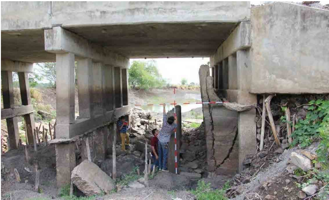
Photo 8.1-5 The measurement of riverbed scour, existing abutment and pier
