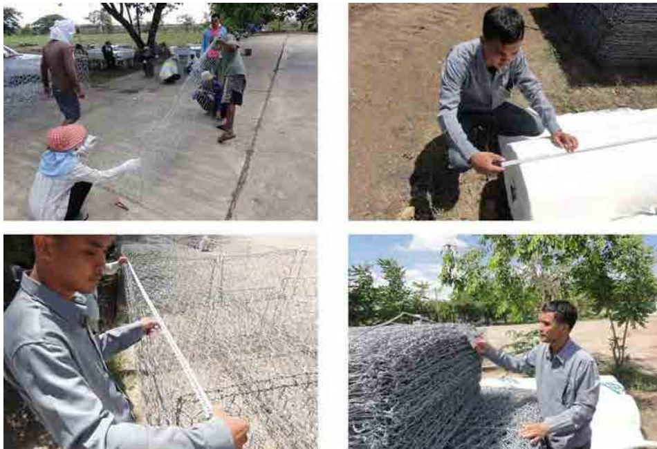
Photo 8.1-11 Material inspection of gabion works performed by BRR staff
