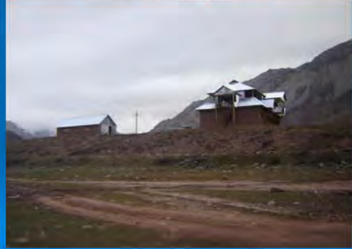
New office of Beekeeping Support Center, square 242 sq. m, built by people of the region, migrants families by the method of "Hashar" view from Khingob river side
