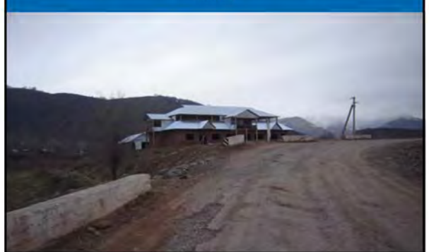
New office of Beekeeping Support Center, square 242 sq. m, built by people of the region, migrants families by the method of "Hashar"
