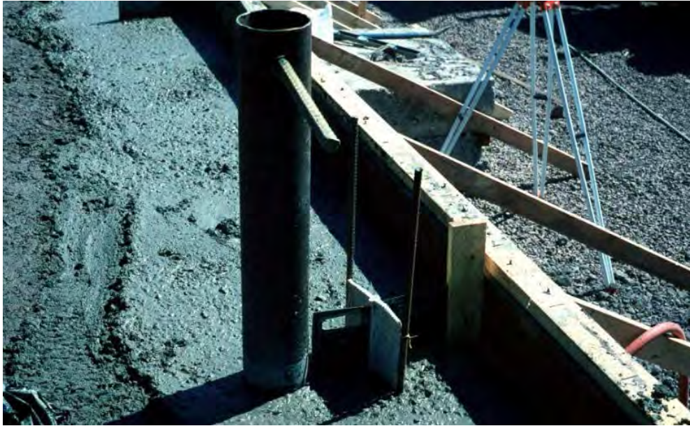
Fig 7.3-16 Installation of waterstop, joint drain, and crack initiator
