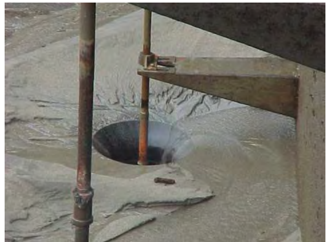
Fine particles discharged through bottom gates
