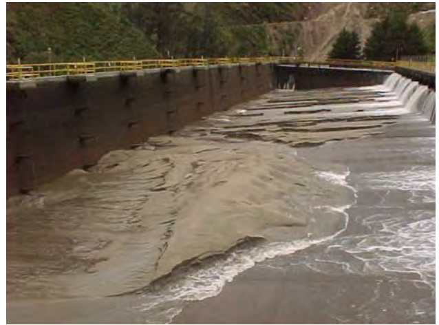
Washing away sediment remaining at the bottom of the settling basin
