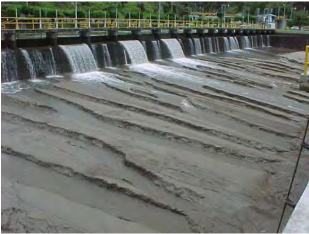
Washing away sediment remaining at the bottom of the settling basin
