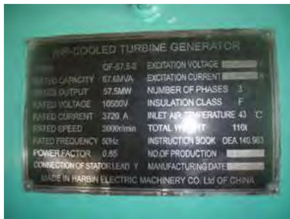
Figure 19- 2 Sample rating plate of generator
