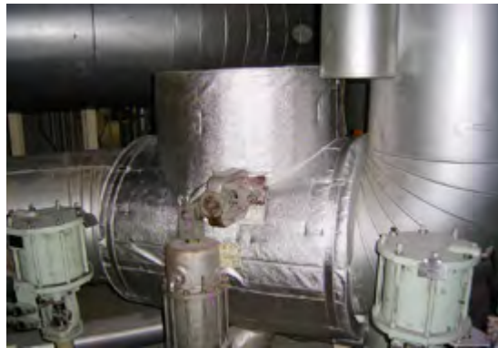
Photo 167-1 Extraction non-return valve
