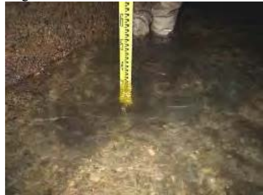
Erosion of lining concrete
