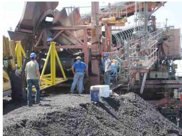
Photo 167-a2-5 Replacement of bucket wheel drive
