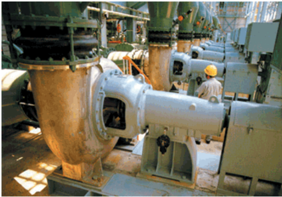
Photo 167-a8-10 Inspection of desulfurization pump
