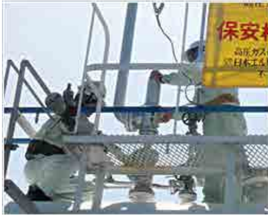
Photo 167-a5-1 Inspection of safety valve
