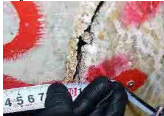
Cracks in lining concrete
