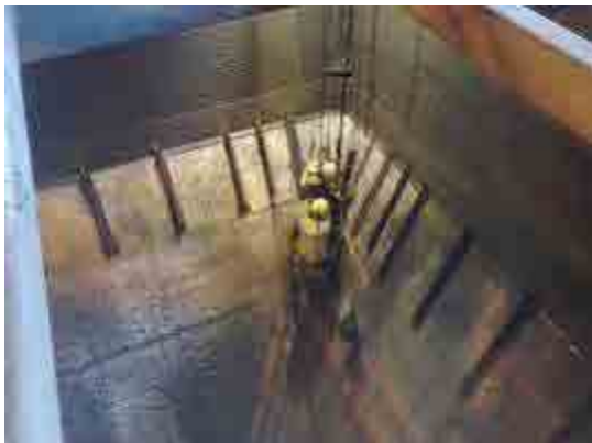
Photo 167-a2-8 Inspection of coal bunker lining
