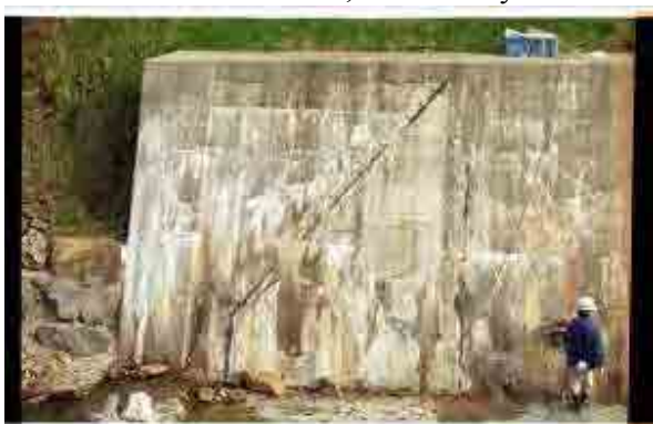
Alkali aggregate reaction
