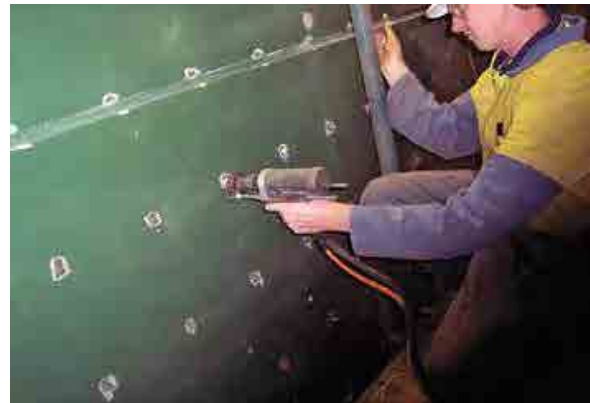
Photo 167-a2-9 Lining of coal bunker
