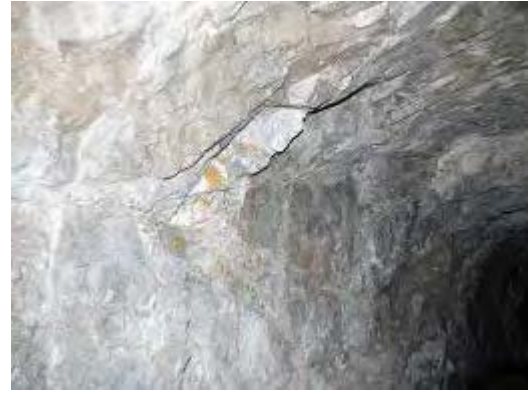
Rockfall from tunnel surface
