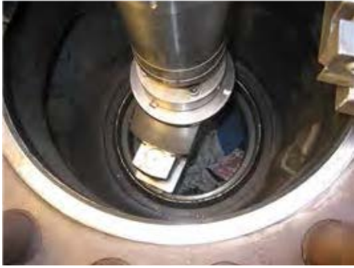
Photo 162-22 Repair of MSV seat
