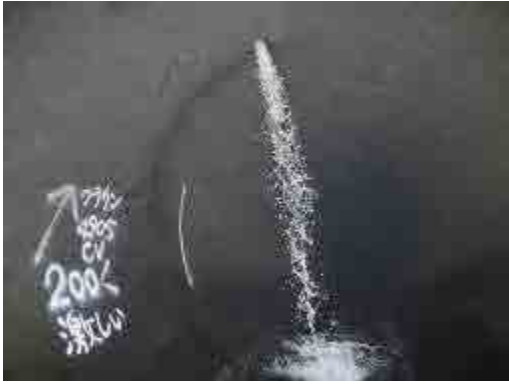
Water leakage from lining concrete
