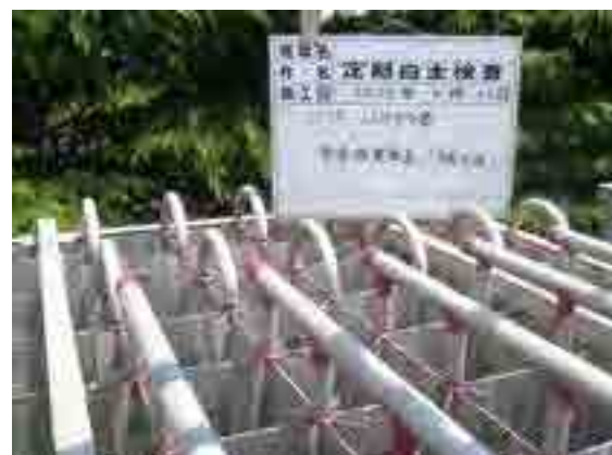
Photo 167-a5-3 Open inspection of air fin vaporizer
