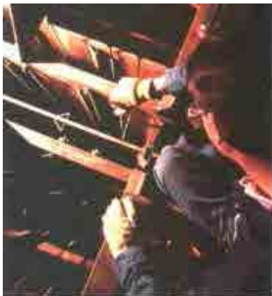
Photo 167-a8-4 Inspection of dust collection plate
