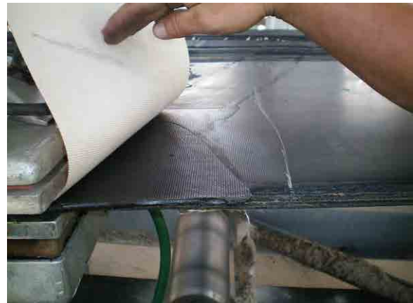
Photo 167-a2-7 Repair of belt conveyor
