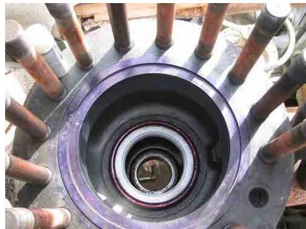
Figure 162-6 Repair of MSV seat
