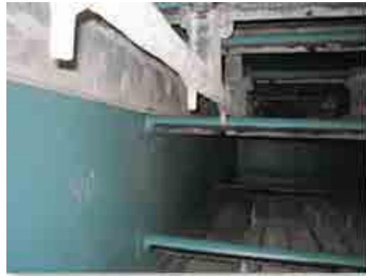
Photo 167-a8-11 Flake lining de-sox dust removal tower
