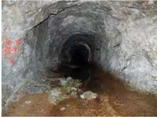
Rockfall from tunnel surface
