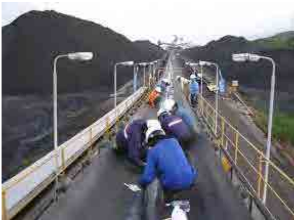
Photo 167-a2-7 Repair of belt conveyor
