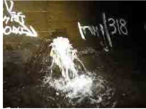
Water leakage from lining concrete
