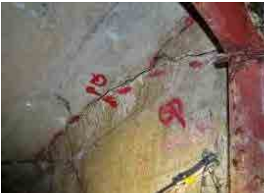
Cracks in lining concrete
