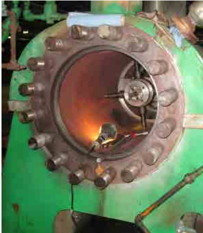
Photo 161-1 Inspection of BFP internal
