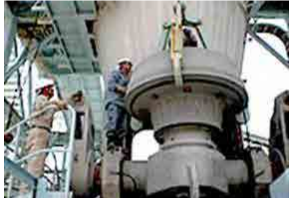
Photo 167-a2-15 Removal of roller tire
