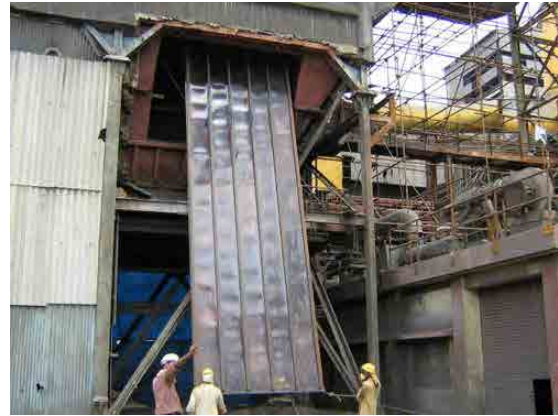
Photo 167-a8-3 Replacement of dust collection plate
