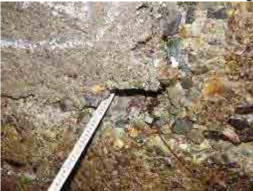
Erosion of lining concrete
