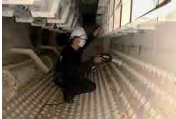
Photo 160-2 Inspection of drum internal
