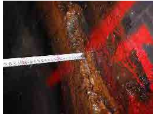
Difference in level of lining concrete
