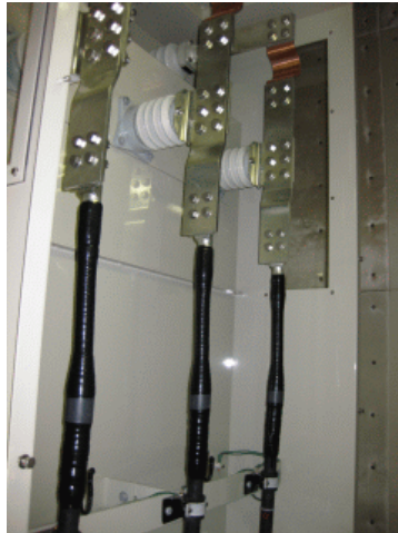
Figure 90 Application examples of flexible conductors
