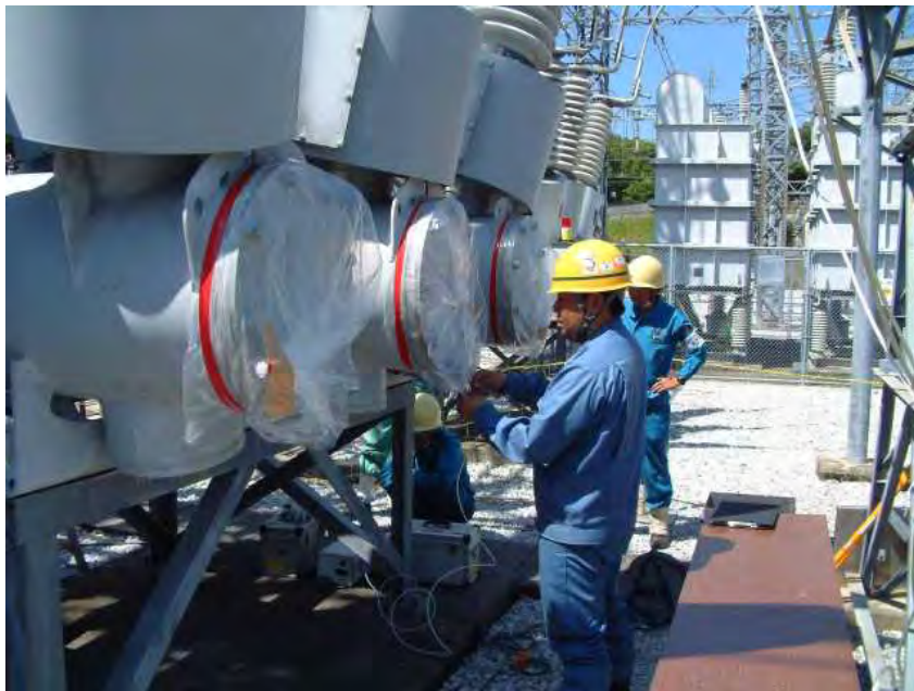
Figure 125 Accumulation method for gas leakage test
