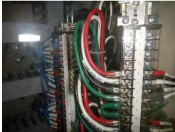
Figure 143 Terminal connection example (Japanese example)
