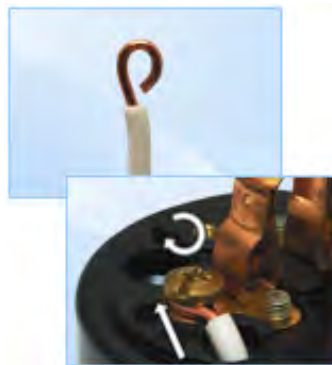
Figure 142-2 Wrap tightening example
