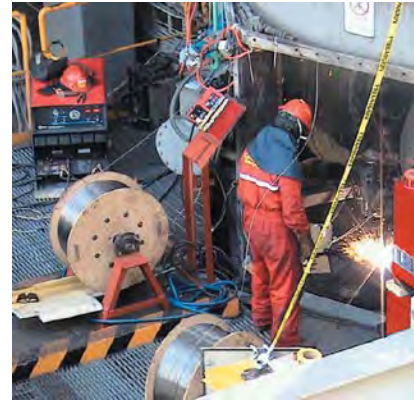
Photo- 16: Hard-facing of roller table
