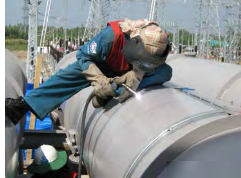
Photo- 24: Aluminum welding of IPB
