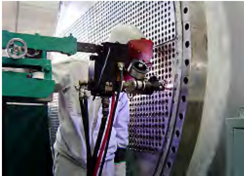
Photo- 23: Titanium seal welding of tube
