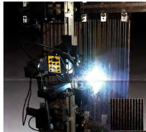
Photo- 18: Overlay welding of boiler furnace wall
