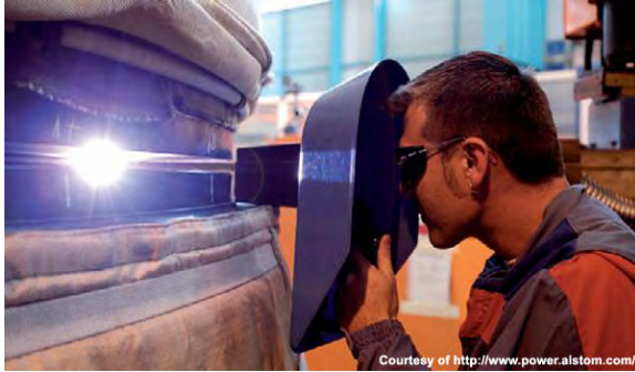
Photo- 19: Laser welding of gas turbine rotor (ALSTOM)
