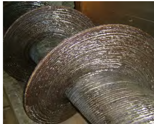
Photo- 12: Hard-facing repair of screw conveyor
