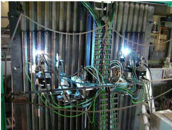
Photo- 17: Overlay welding of incineration boiler
