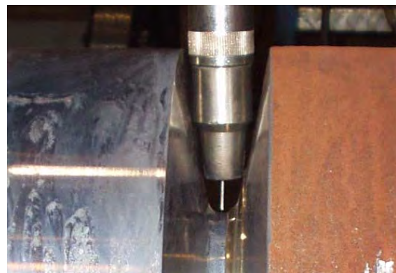
Photo- 6: Welding of heavy wall piping
