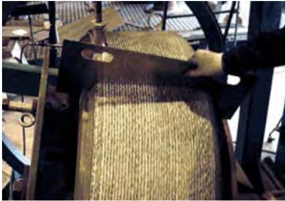
Photo- 15: Repair welding of roller tire
