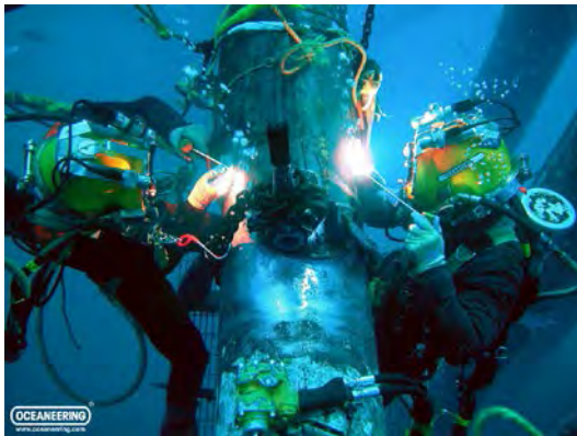
Photo- 21: Divers welding subsea pipeline
