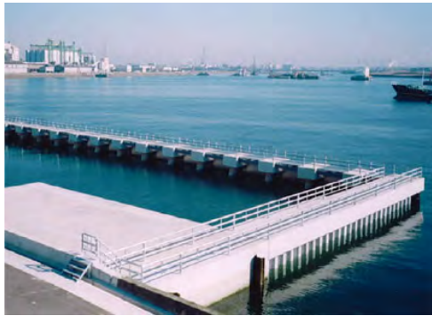
Photo- 8: Curtain wall intake facility
