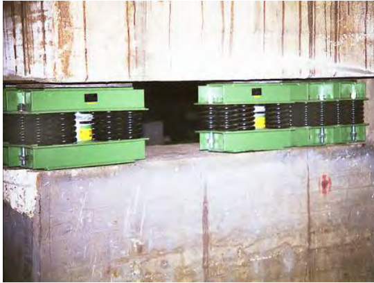
Photo- 6: Coal mill spring mount
