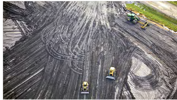
Photo- 44: Landfilling by ash
