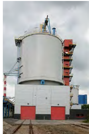
Photo- 20: Fly-ash silo
