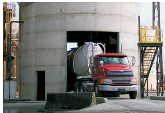
Photo- 30: Fly-ash loading facility
