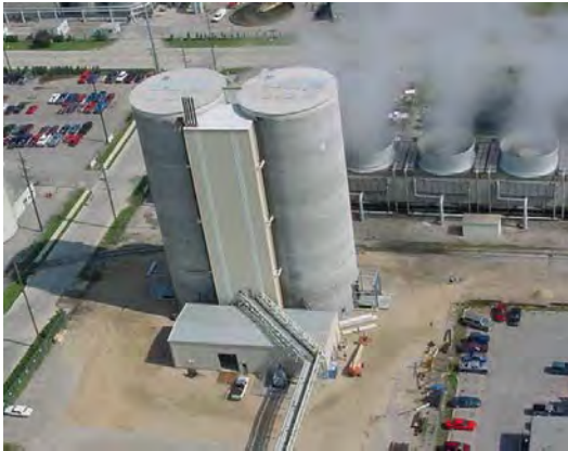
Photo- 19: Fly-ash silo
