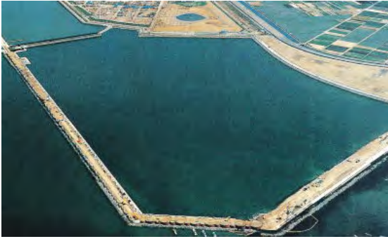
Photo- 39: Ash Disposal Pond
