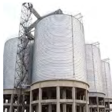
Photo- 24: Fly-ash silo
