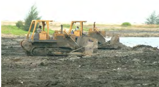
Photo- 45: Landfilling by ash
