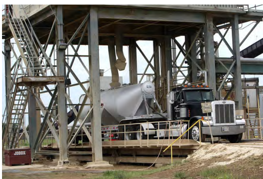
Photo- 29: Fly-ash loading facility
