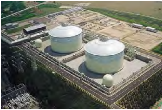
Photo- 36: Protection dike
