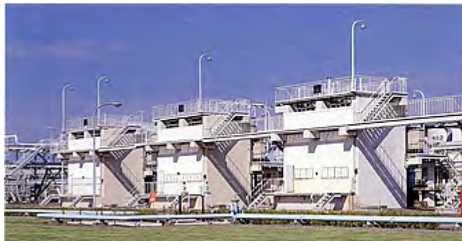
Photo- 46: Sea water type vaporizer
