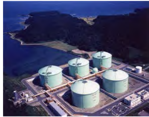
Photo- 37: Protection dike
