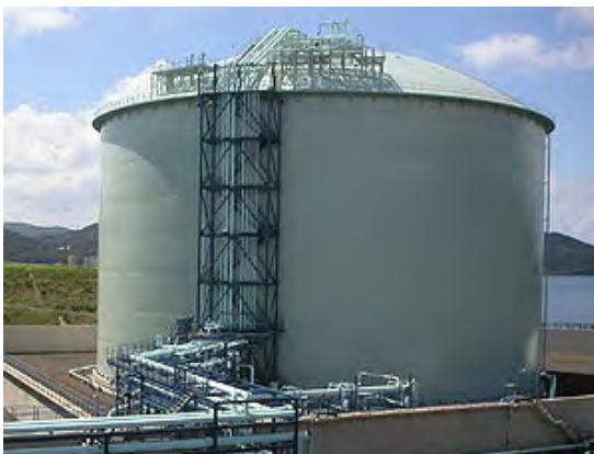
Photo- 28: Low temp. double hull LPG tank
