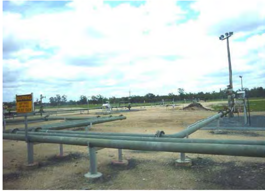
Photo- 37: Reactor (Link energy)
