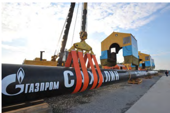
Photo- 35: Welding house
