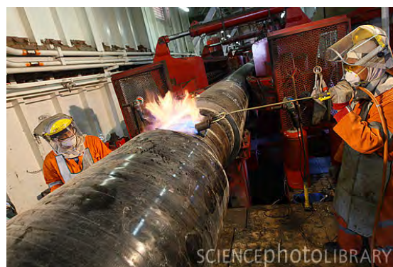
Photo- 24: Welding of off-shore pipeline
