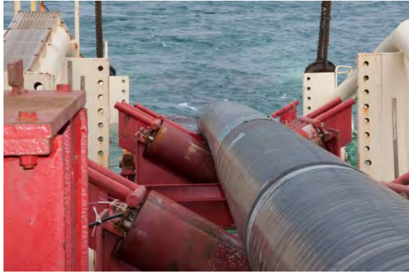
Photo- 25: Laying off-shore pipeline
