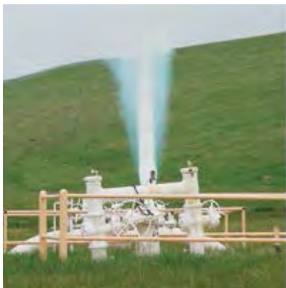
Photo- 17: Purging of gas pipeline
