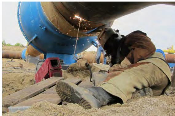
Photo- 30: Arc welding of pipeline on the land http://www.gazprom.com/press/news/2011/july/article115149/
