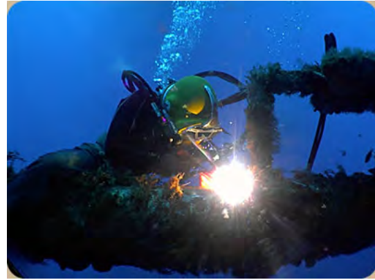
Photo- 26: Welding of subsea pipeline
