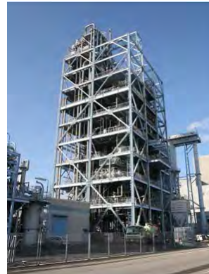
Photo- 41: Coal gasification plant
