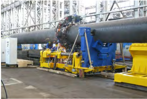
Photo- 33: Flash butt welding
