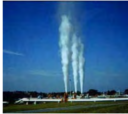
Photo- 16: Purging of gas pipeline
