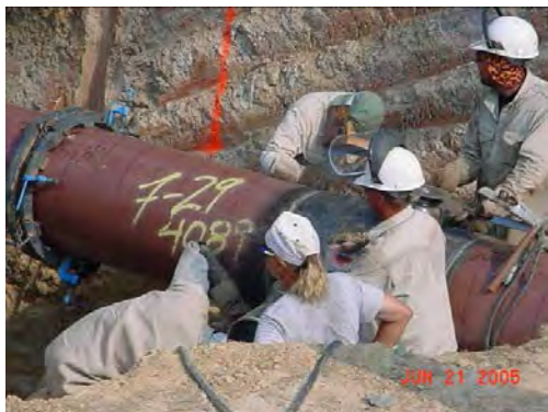
Photo- 29: Arc welding of buried pipeline http://teeic.anl.gov/er/transmission/activities/act/index.cfm
