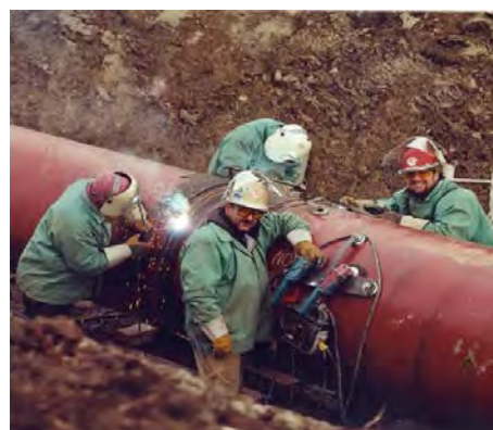
Photo- 32: Arc welding http://rattlestan.com/projects.html
