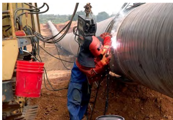
Photo- 31: Mig welding http://www.indiazooms.com/?p=2896
