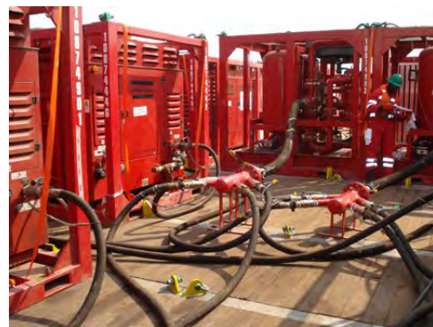
Photo- 28: Compressor for pressure test
