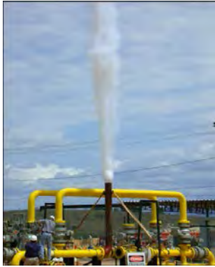
Photo- 15: Purging of gas pipeline
