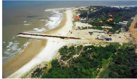
Photo- 3: Natural gas pipeline in Nam Con Son
