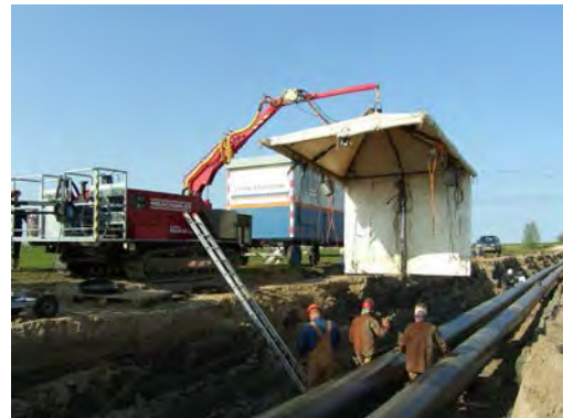
Photo- 36: Welding tent
