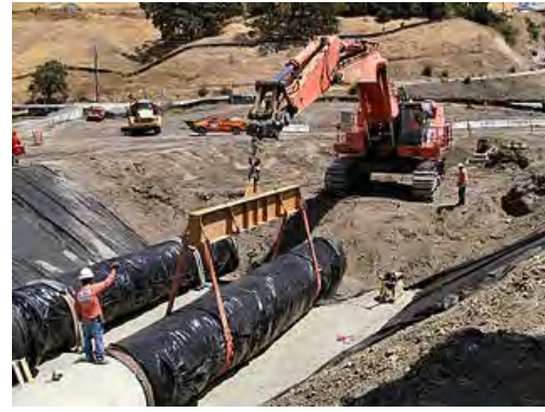
Photo- 74: Buried pipeline under the road
