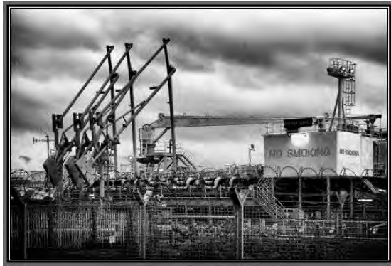
Photo- 11: Tanker wharf keep out fence
