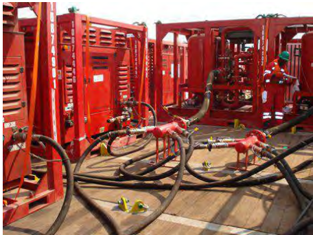
Photo- 86: Compressor for pressure test
