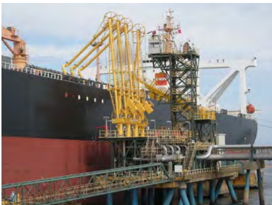
Photo- 7: Oil unloading facility
