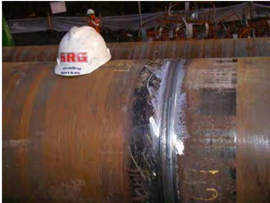
Photo- 46: TIG welding
