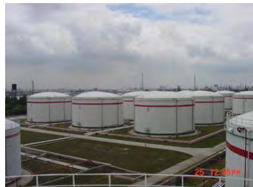
Photo- 106: Outdoor oil storage tank
