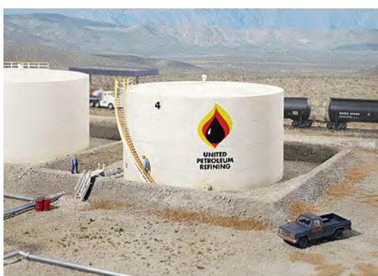
Photo- 125: Oil tank dike
