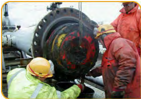
Photo- 102: Cleaning pig
