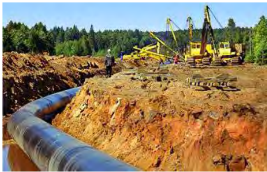
Photo- 62: Underground pipeline
