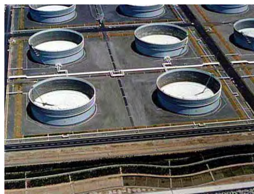
Photo- 126: Oil tank dike
