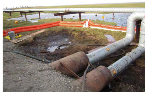
Photo- 78: Sheath tube for pipeline under the road
