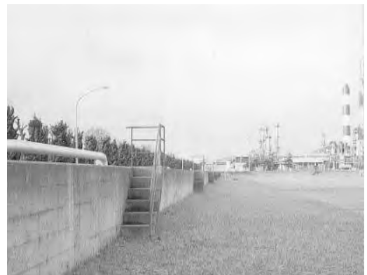
Photo- 129: Oil tank dike
