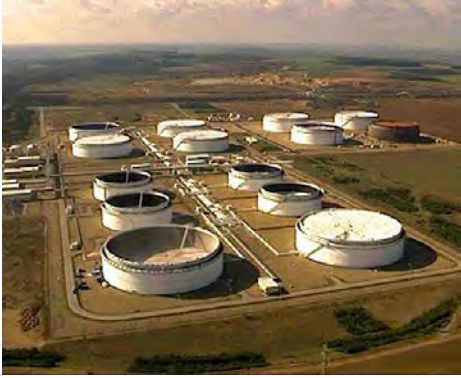
Photo- 107: Specific oil storage tank
