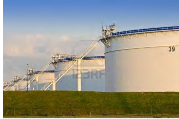
Photo- 108: Specific oil storage tank
