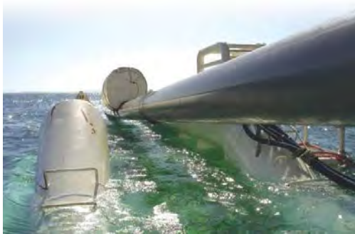
Photo- 52: Coated offshore pipeline
