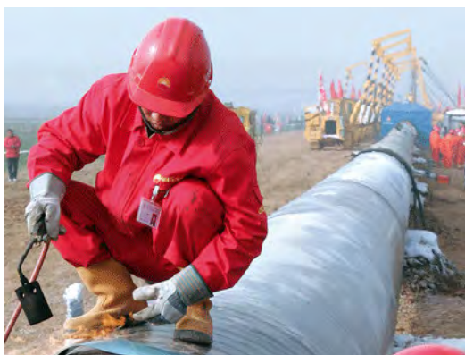
Photo- 54: Corrosion protection taping
