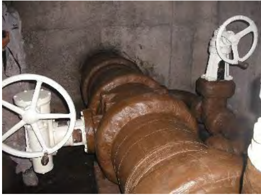
Photo- 56: Corrosion protection taping
