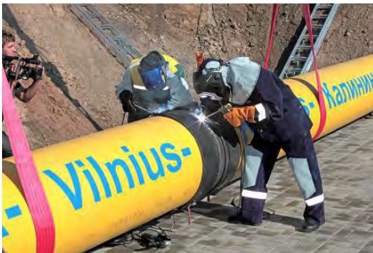
Photo- 48: Arc welding
