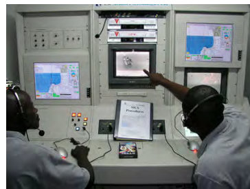
Photo- 91: Pipeline monitoring
