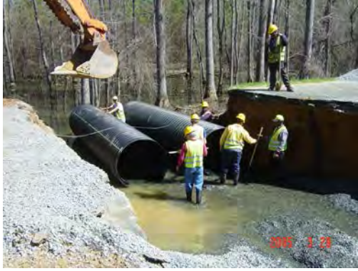
Photo- 73: Buried pipeline under the road
