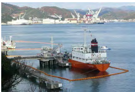
Photo- 123: Oil fence
