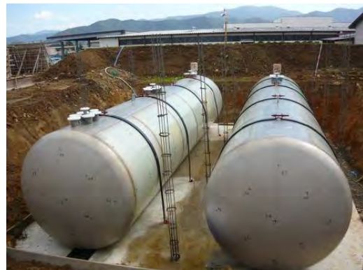
Photo- 111: Underground oil storage tank
