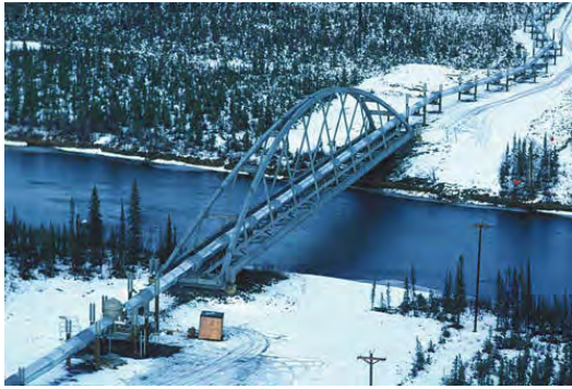
Photo- 76: Pipeline river crossing
