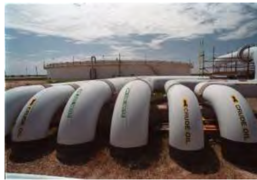
Photo- 63: Underground pipeline
