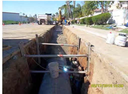
Photo- 66: Pipeline buried under road
