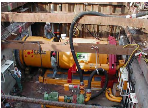
Photo- 67: Pipeline under railroad
