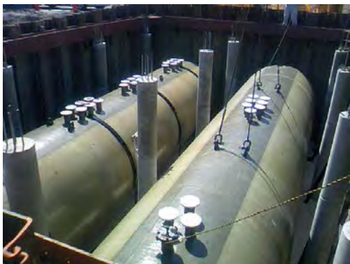
Photo- 110: Underground oil storage tank
