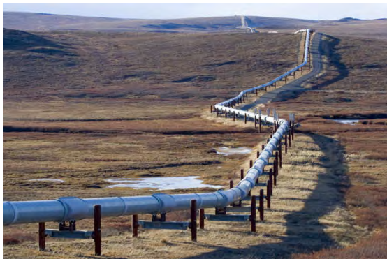
Photo- 60: Pipeline on the ground
