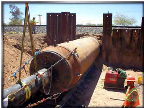
Photo- 75: Pipeline below railroad
