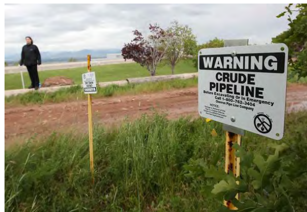
Photo- 64: Underground pipeline
