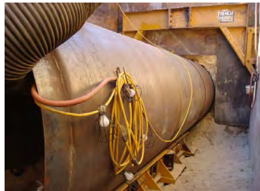
Photo- 68: Sheath tube under railroad
