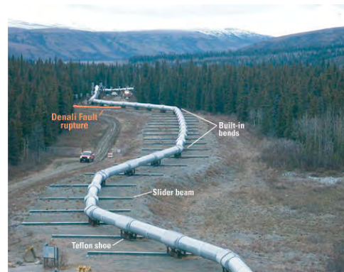
Photo- 61: Pipeline on the ground
