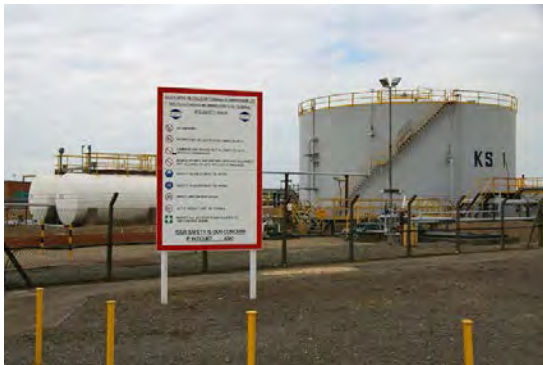
Photo- 121: Fence and warning around oil tank
