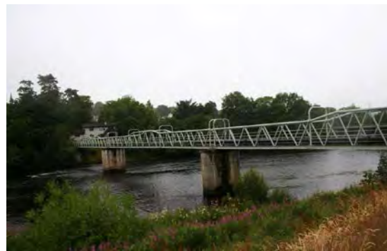
Photo- 77: Pipeline river crossing
