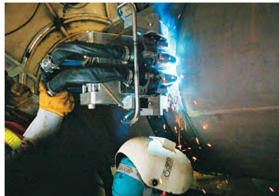
Photo- 49: MIG welding
