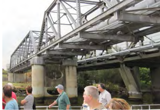
Photo- 80: Piping bridge
