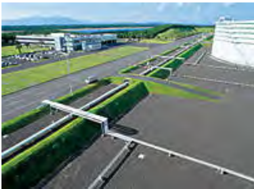
Photo- 128: Oil tank dike
