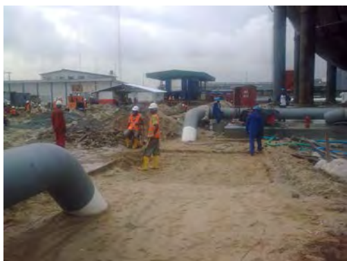
Photo- 72: Road crossing pipeline
