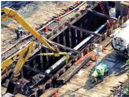
Photo- 65: Pipeline buried under road
