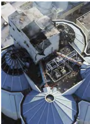
Photo- 77: Coal dust explosion of silo
