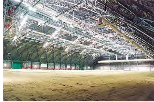
Photo- 80: Gable type indoor coal storage yard
