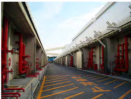
Photo- 52: Coal yard fire fighting piping
