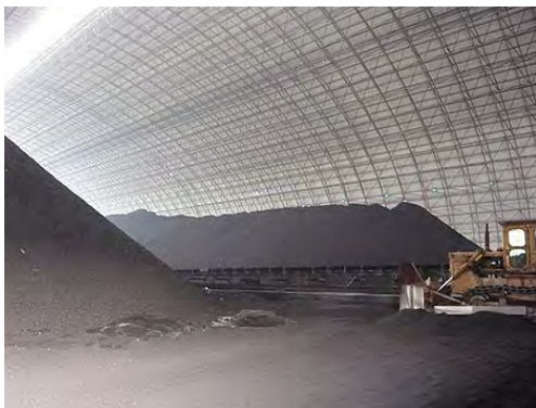
Photo- 81: Gable type indoor coal storage yard
