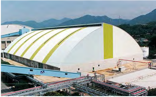
Photo- 79: Gable type indoor coal storage yard
