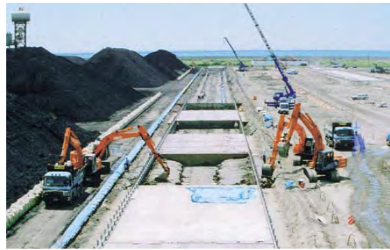
Photo- 74: Foundation of reclaimer roadbed
