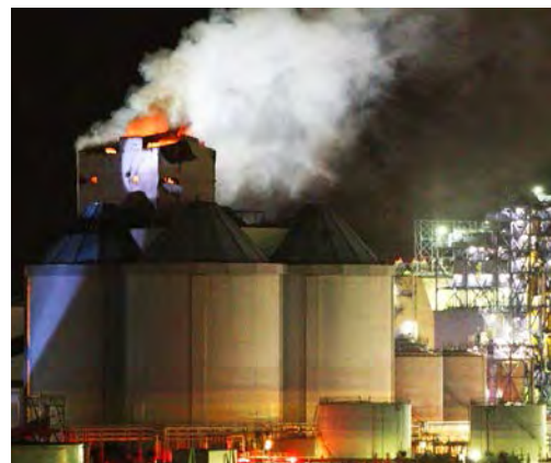
Photo- 78: Coal dust explosion of silo
