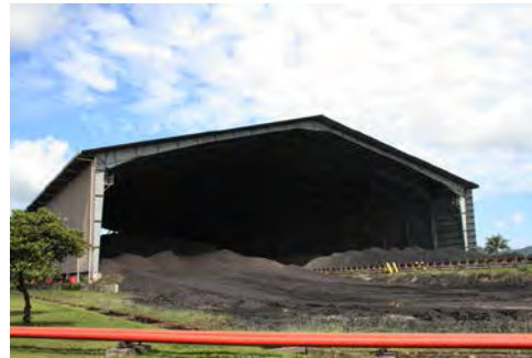
Photo- 82: Gable type indoor coal storage yard
