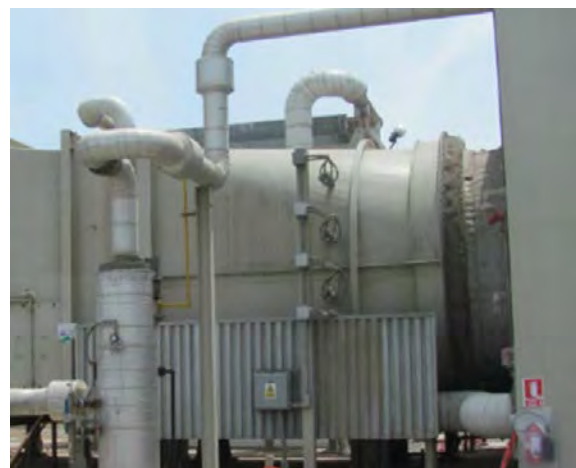
Photo- 40: Exhaust diffuser
