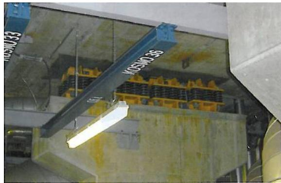
Photo- 25: Application of elastic support for steam turbine bed
