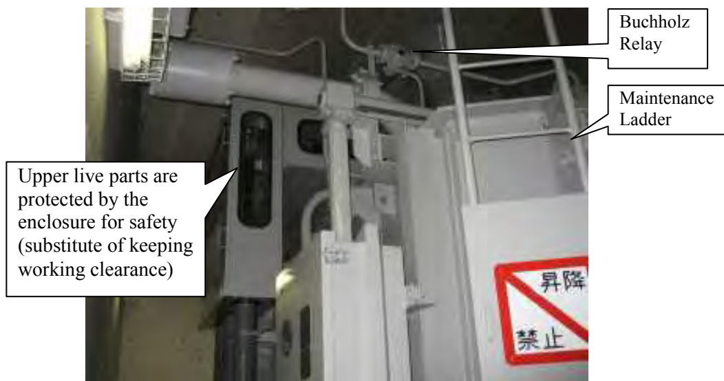
Figure 390-2 Installation example of maintenance ladder (Japanese case)
