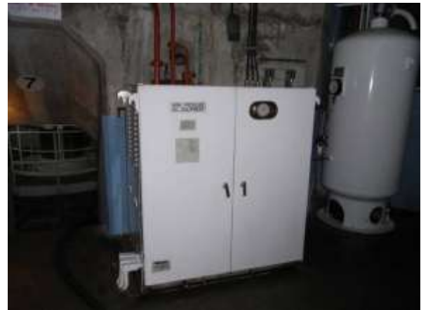
Source: Prepared by the Survey Team
