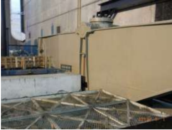
Source: Prepared by the Survey Team
