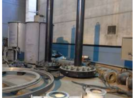
Source: Prepared by the Survey Team
