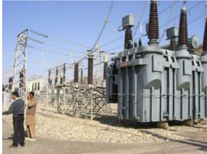
Source: Prepared by the Survey Team
