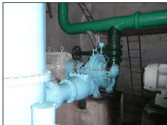
Photo 4-7 Standby Cooling Pumps for Units 1 to 4
