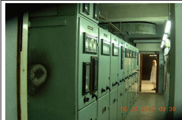
Photo 4-17 11 kV Station Service Cubicles
