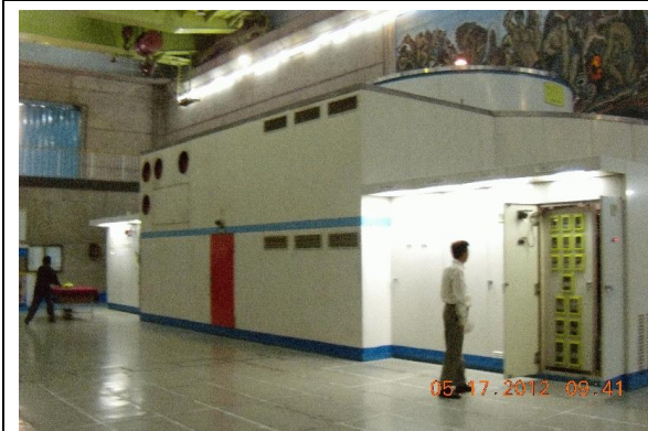
Photo 4-15 Governor and AVR Cubicle for Unit 1
