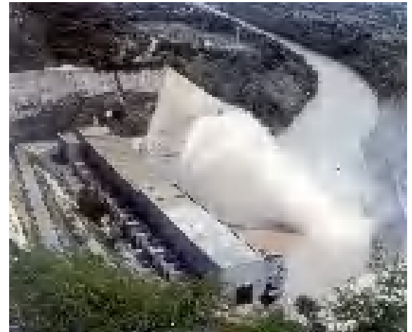
Source: Mangla Power Station Presentation File "Briefing for JICA on February 28, 2012.pptx"
