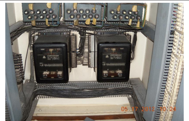
Photo 4-16 Generator Protection Relay
