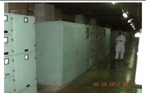
Photo 4-18 400 V Station Service Cubicles
