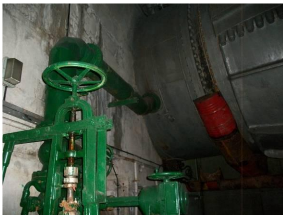
Photo 4-6 Cooling Water Supply System
