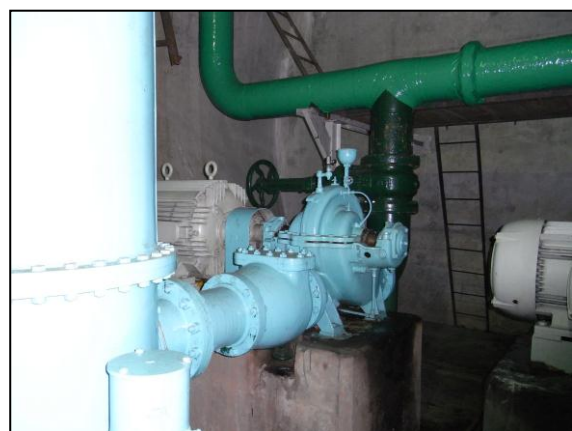
Photo 4-7 Standby Cooling Pumps for Units 1 to 4
