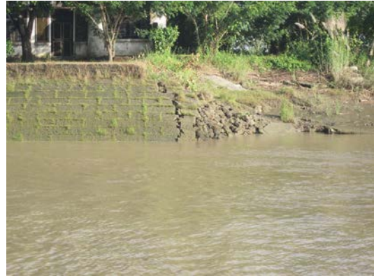
Figure 5.4.3: Twante Area Embankment Damage
