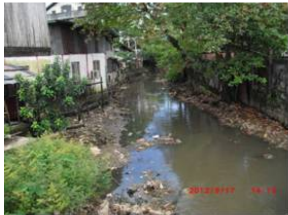
Shwehle Chaung Drainage Channel (No.20)
