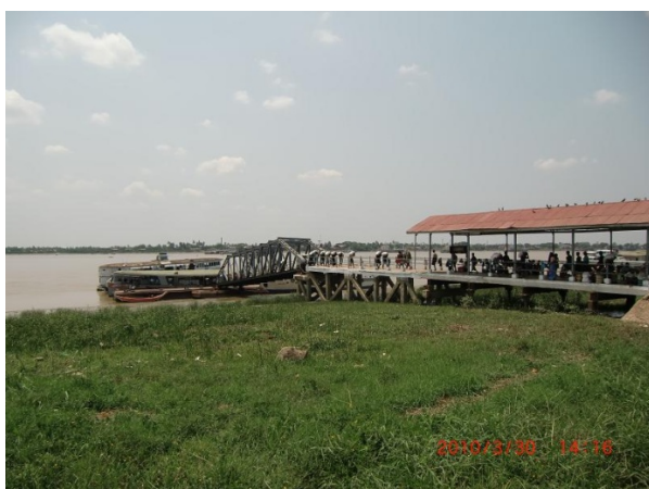
Jetty at Botahtaung Area
