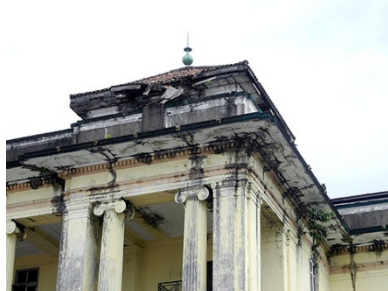
Roof damaged by strong winds
