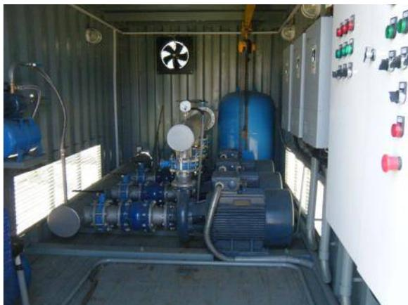
Picture 7-5: booster pump for pipeline
