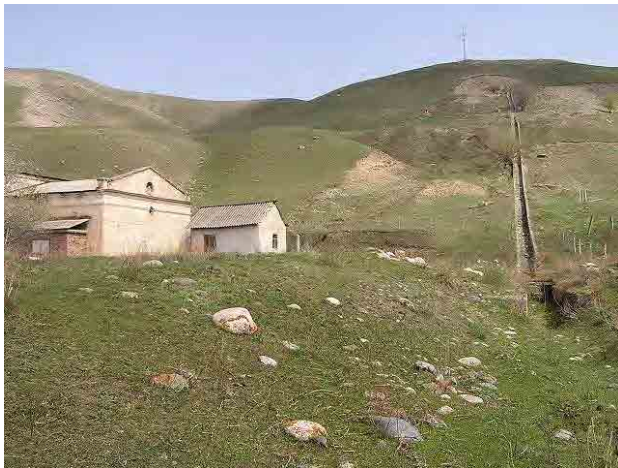
Photo 6-2-54: Powerhouse and Spillway from Head Tank
