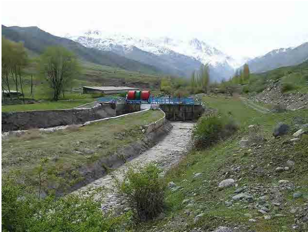
Photo 6-2-101: Existing Intake for Irrigation near Ak Suu-1 Intake
