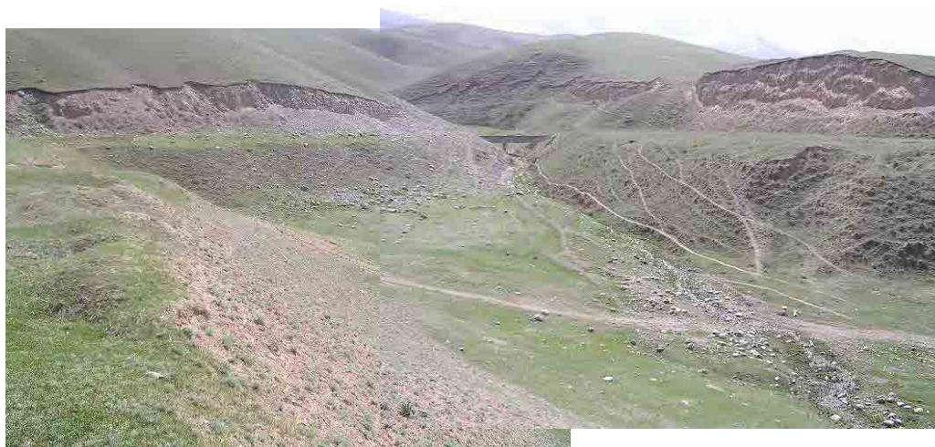
Photo 6-2-62: Headrace and Aqueduct
