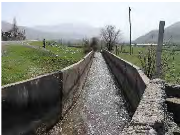
Photo 6-2-89: Irrigation Canal near No.2 Site
