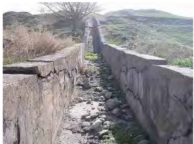
Photo 6-2-50: Spillway from Head Tank
