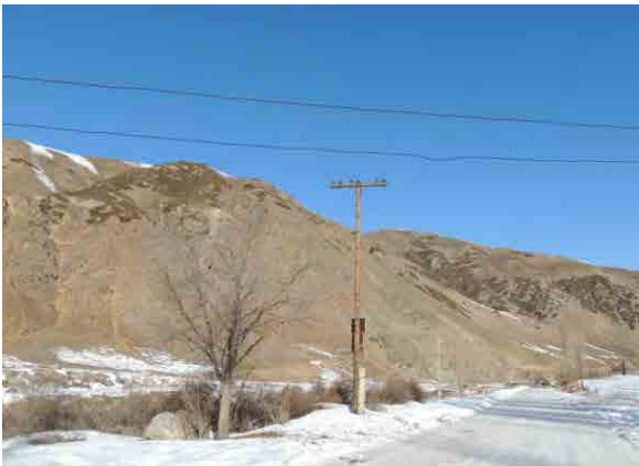
Photo 6-2-53 10kV Distribution Line for Local Power Supply
