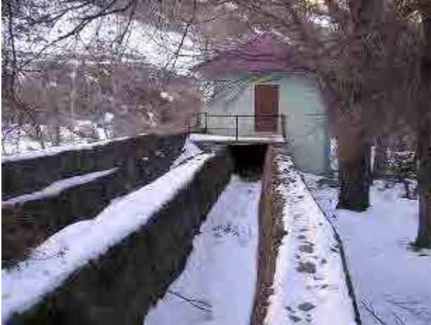
Photo 6-2-49: Cut Slope above Headrace
