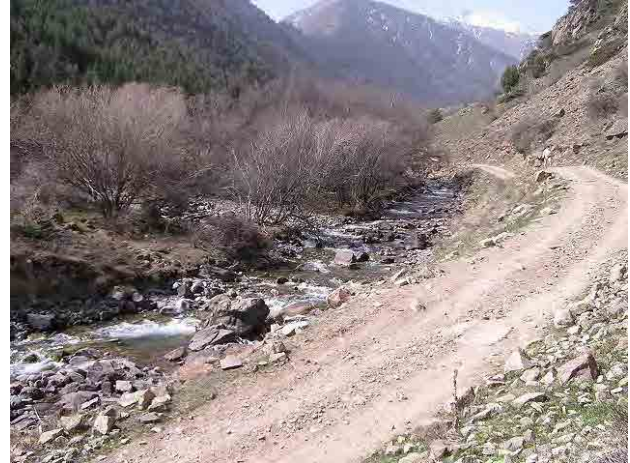
Photo 6-2-82: No.1 Intake Site and Road
