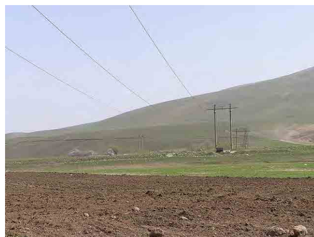
Photo 6-2-92: 220kV Transmission Line near No.2 Powerhouse
