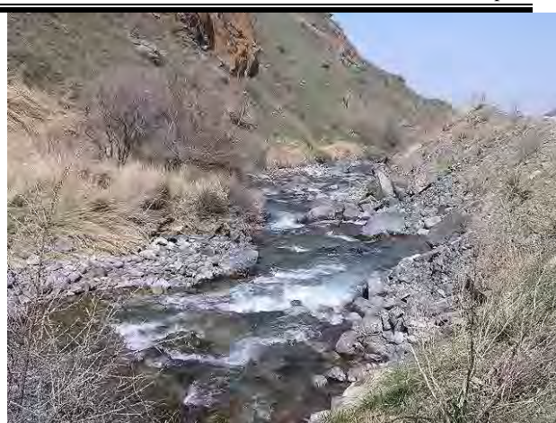
Photo 6-2-86: No.2 Intake (downstream)
