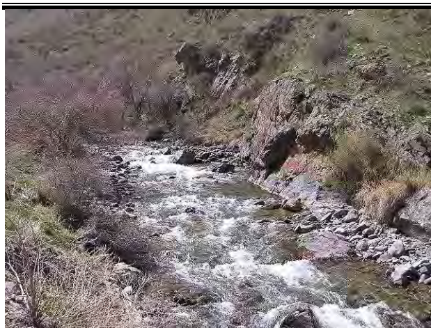
Photo 6-2-85: No.2 Intake Site (upstream)
