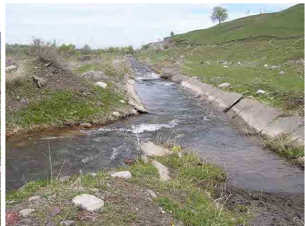
Photo 6-2-105: Headrace for Captive Power
