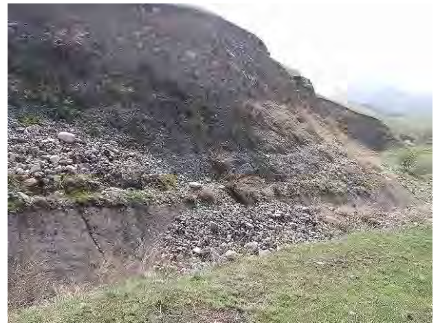
Photo 6-2-61: Headrace Buried with Soil
