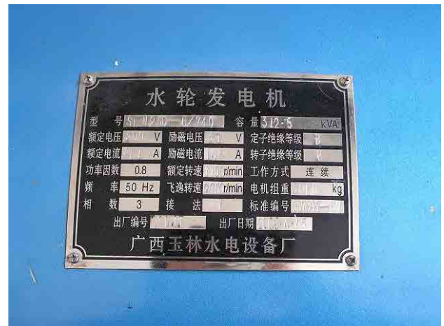
Photo 6-2-111: Generator Nameplate for Captive Power
