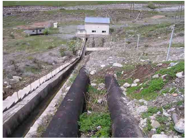
Photo 6-2-109: Powerhouse for Captive Power
