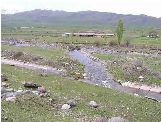
Photo 6-2-104: Intake for Captive Power
