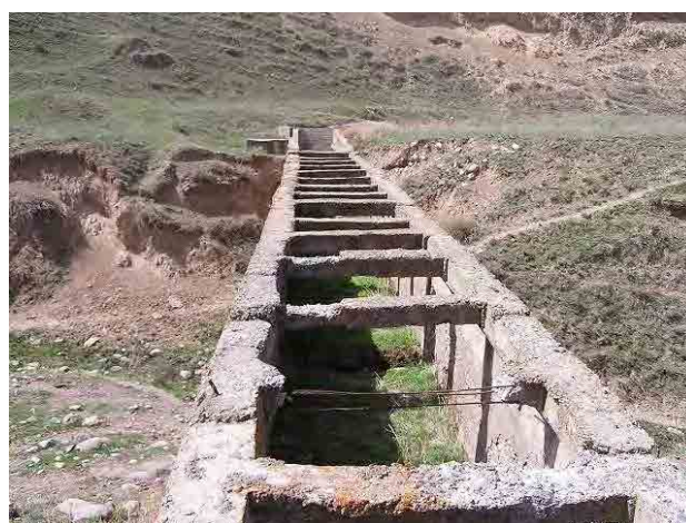
Photo 6-2-64: Aqueduct (2 m x 2 m)
