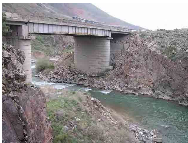
Photo 6-2-97: Road Bridge downstream of Chon-Kemin-3 Intake Site
