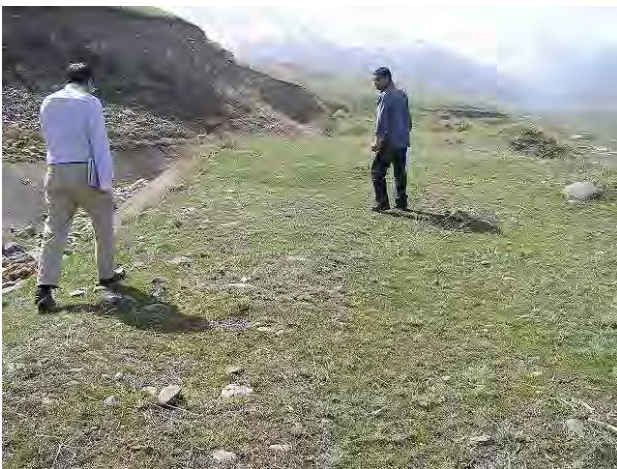
Photo 6-2-60: Platform for Headrace (10 m wide)
