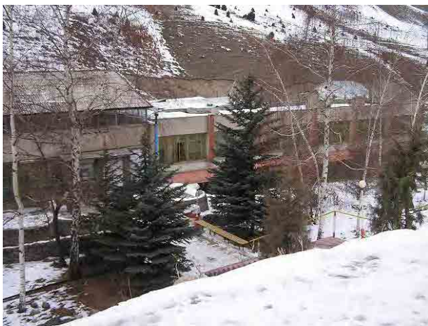
Photo 6-2-75: Spa Resort Building
