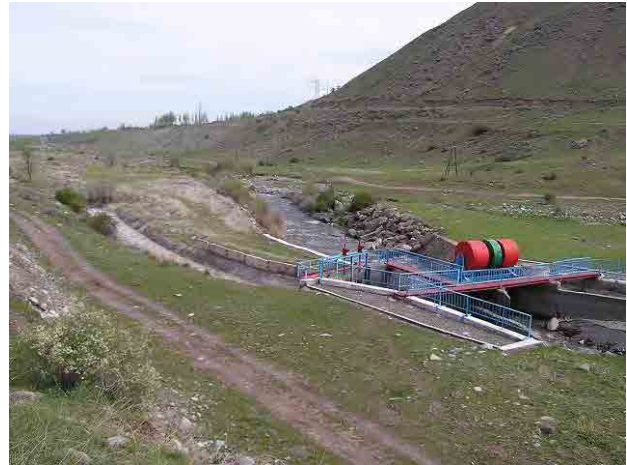
Photo 6-2-102: Existing Intake for Irrigation near Ak Suu-1 Intake
