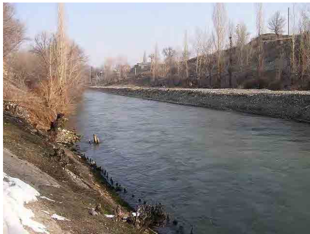
Photo 5-7-14: Excavated Tailrace
