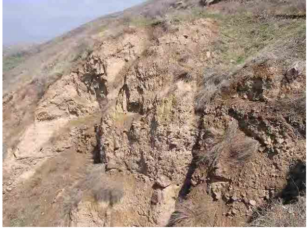
Photo 6-2-36: Cut Slope above headrace
