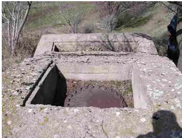
Photo 6-2-28: Manhole & Anchor Block of Penstock
