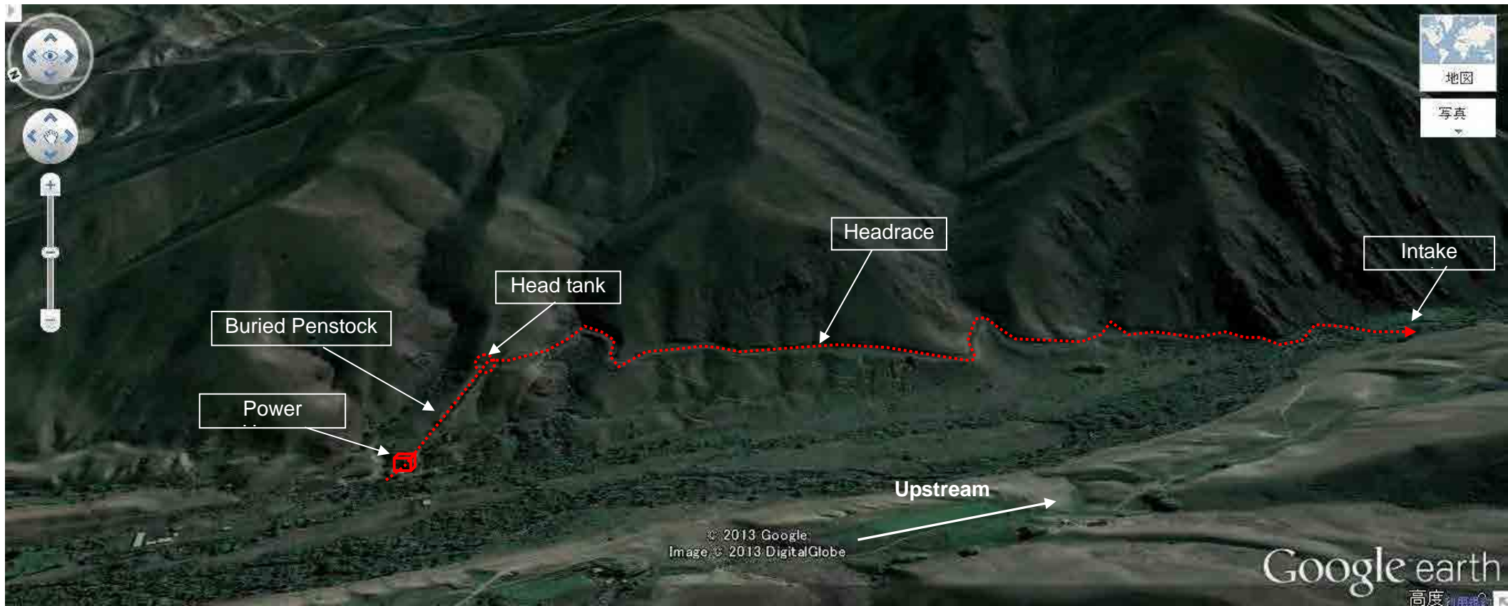
Figure 6-2-10 Bird View for Abolished Djardy-Kainda SHPP (seen from west to east)
