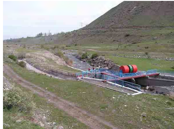
Photo 5-3-2 Irrigation Intake Facility at Ak Suu River
