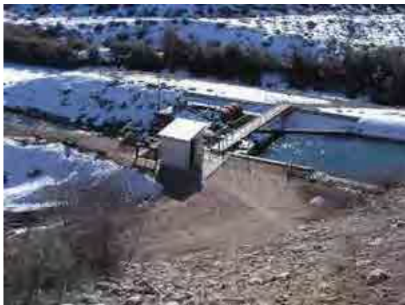
Photo 5-7-1 Intake Weir for Issyk-Ata-1
