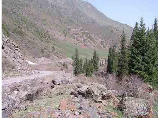
Photo 6-2-12: Upstream of C
