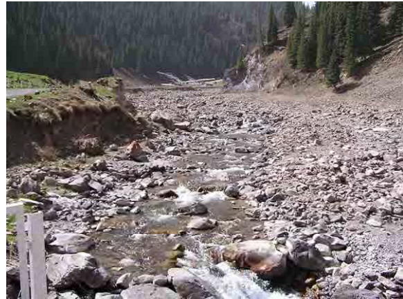
Photo 6-2-2: Upstream from A
