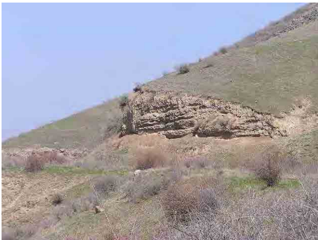
Photo 6-2-41: Cut Slope above Headrace
