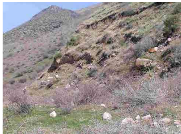
Photo 6-2-42: Cut Slope above Headrace
