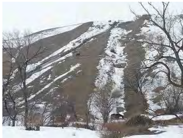
Photo 5-7-8 Slope for Penstock and Spillway from Head Tank
