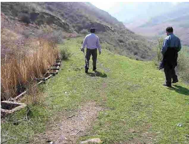
Photo 6-2-33: Platform for Headrace (5 m wide)
