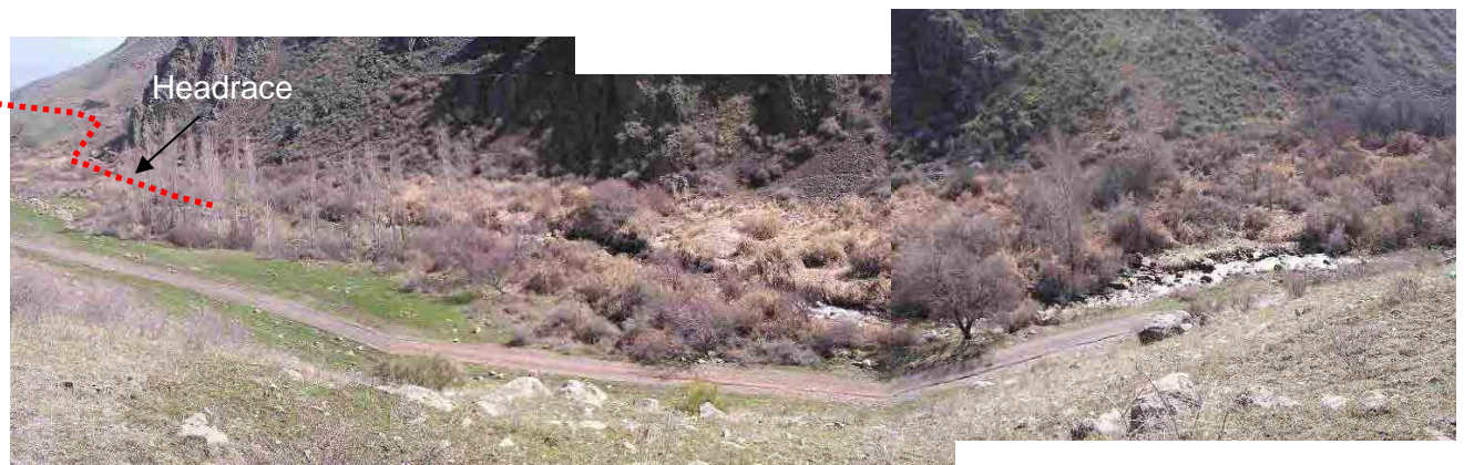
Photo 6-2-43: Intake Site (seen from left bank)
