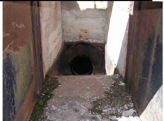
Photo 6-2-31: Inlet of Penstock
