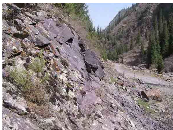
Photo 6-2-5: Slope on roadside between A&B (dip slope)
