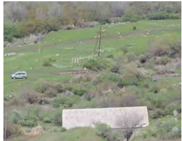
Photo 6-2-47 Positional Relation between 10kV Existing Distribution Line and Old Power Station
