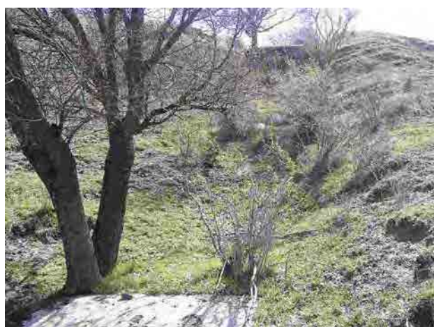
Photo 6-2-24: Slope for Embedded Penstock
