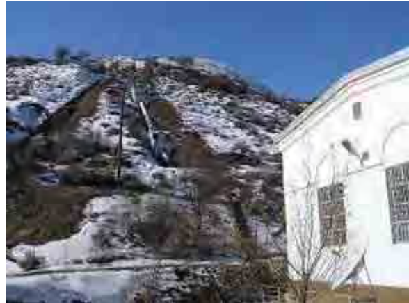
Photo 5-7-4 Issyk-Ata-1 Power Plant (Powerhouse, penstock and spillway from Headtank, seen from right)
