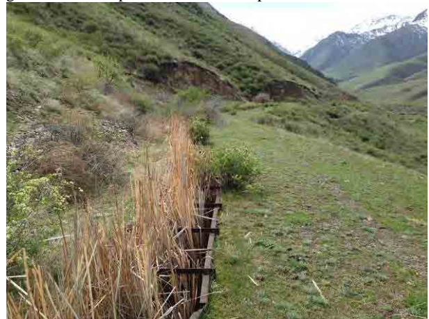
Djardy-Kainda: Old waterway. Part of the waterway remains as it was.
