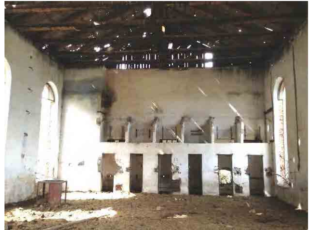
Djardy-Kainda: The inside of the old power house was vacant. Therefore, no waste of old equipment will be generated for disposal in the redevelopment.
