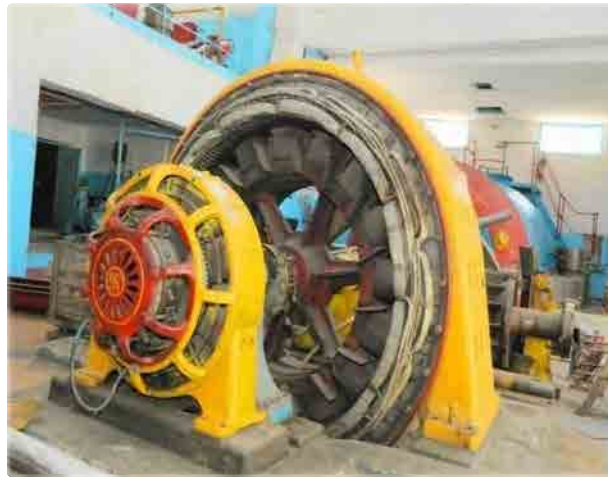
Photo 3-3-1 Generator of Lebedinovka HPP Unit No.2 Stopped by Trouble
