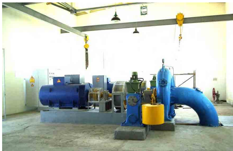
Photo 3-3-2 Water Turbine Generator of Issyk-Ata HPP
