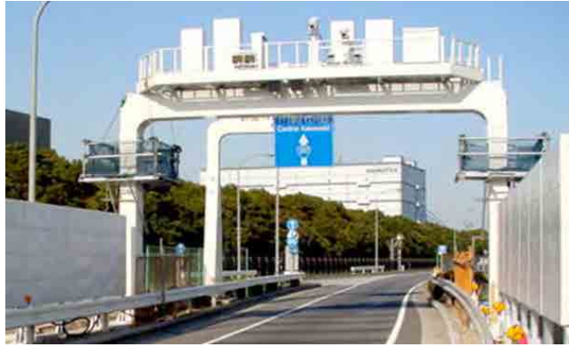
FIGURE 20.1-2 FREE FLOW ETC (ONE LANE AT EXIT)
